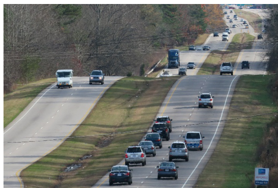
Crests and sags result in poor sight distance.
