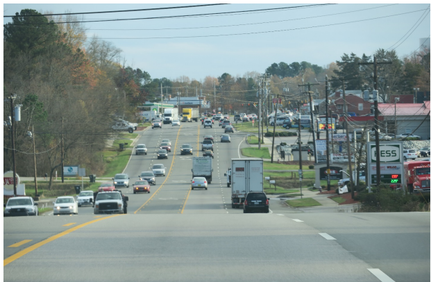
The US 70 typical section varies from five-lanes, including a two-way center turn lane, to a four-lane, median-divided roadway.
