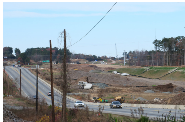
East End Connector construction at the western project terminus
