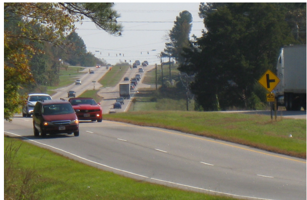
The US 70 typical section varies from five-lanes, including a two-way center turn lane, to a four-lane, median-divided roadway.
