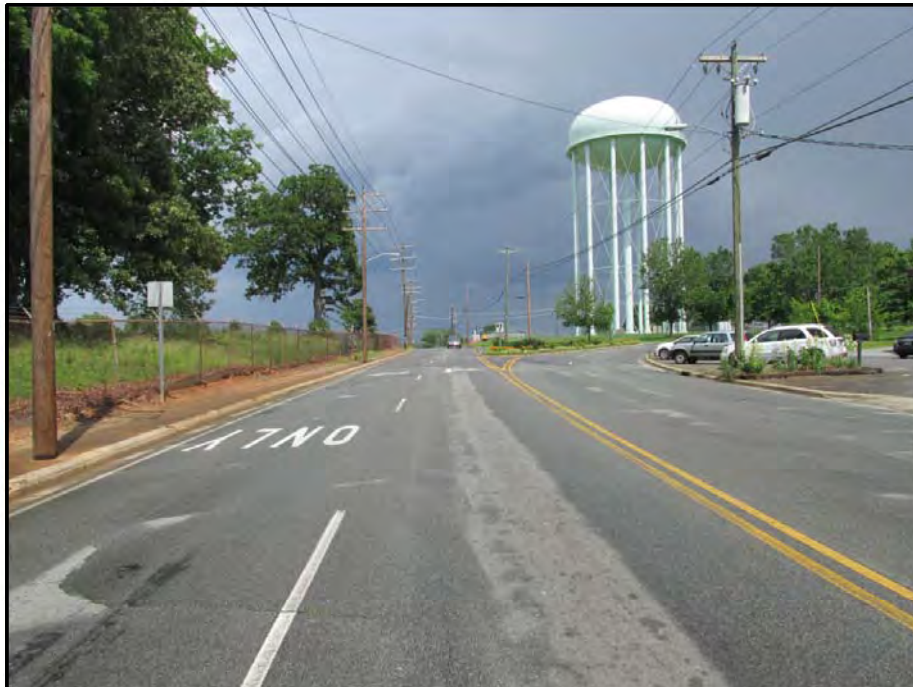
Westbound Approach looking East
