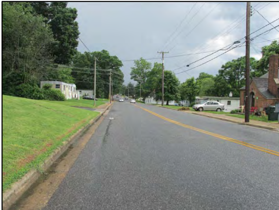
Northbound Approach looking South
