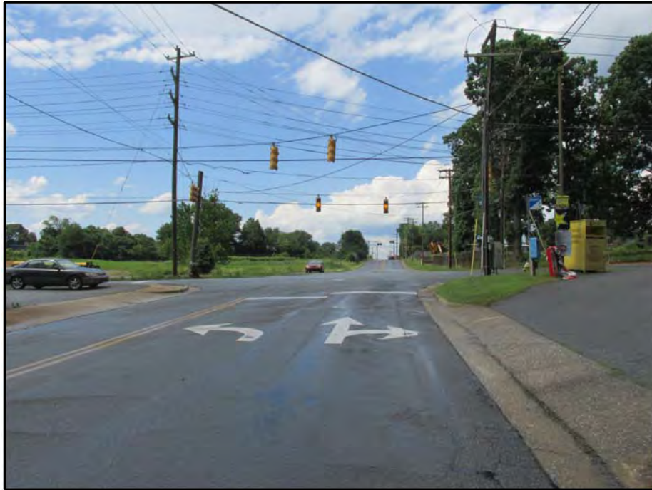
Northbound Approach looking North
