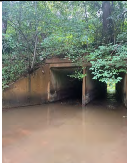
Downstream Structure - Existing 2@ 8'x8' RCBC under Candy Creek Rd.
