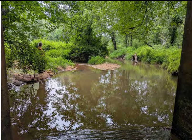
Downstream Structure - Existing 2@ 8'x8' RCBC under Candy Creek Rd.
