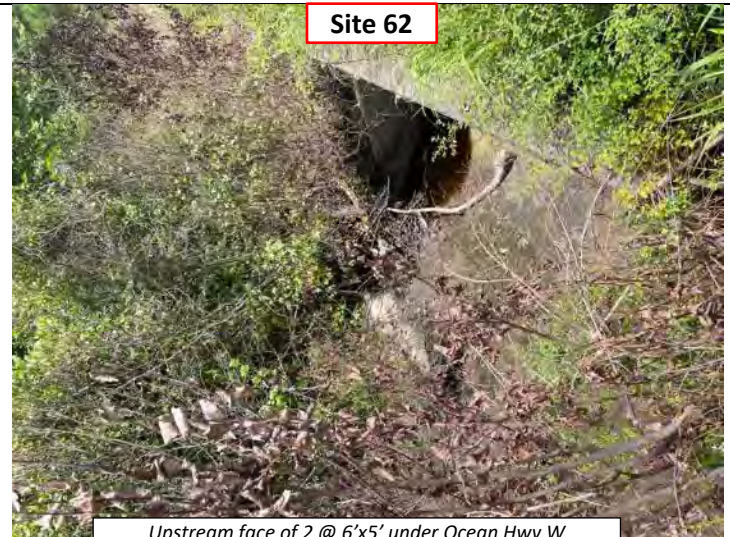
Upstream face of 2 @ 6'x5' under Ocean Hwy W
