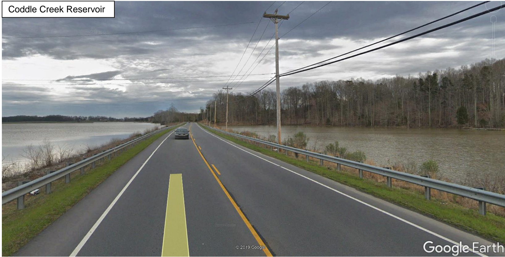
Coddle Creek Reservoir
