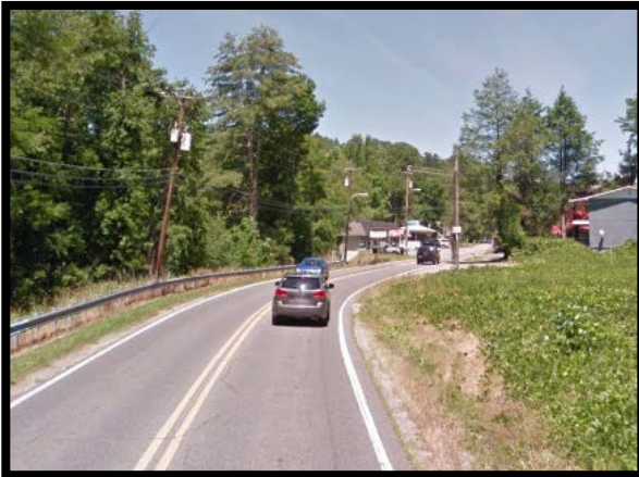
U.S. 19 Headed East, narrow lane width and inadequate shoulders
