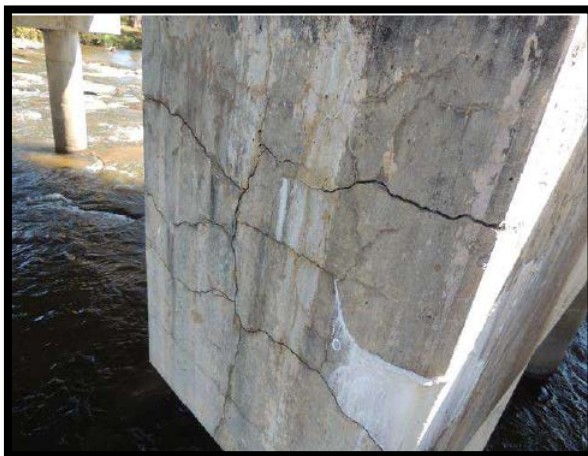
Bridge No. 20 open crack in bent. "Indication of structural deterioration"
