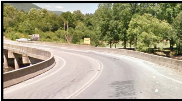
U.S. 19 Headed Approach to Bridge No. 20 over the Tuckasegee River, narrow lane width and inadequate shoulders, limited sight distance
