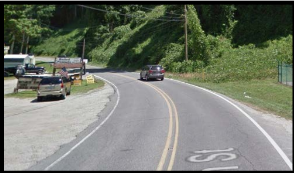
U.S. 19 Headed East, narrow lane width and inadequate shoulders, limited sight distance
