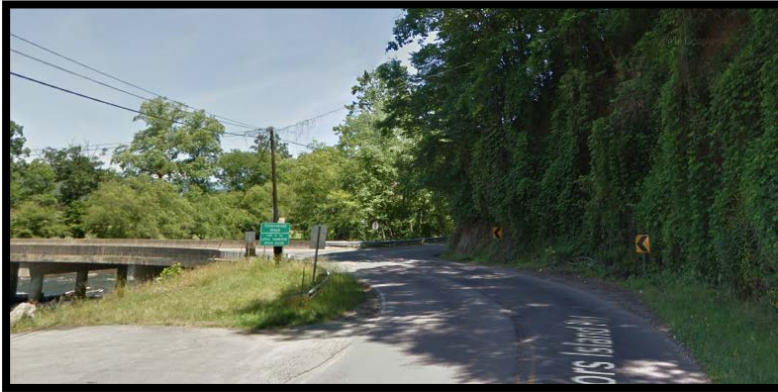
Bridge No. 20, Sharp Horizontal Curve on Bridge narrow lane width and inadequate shoulders, limited sight distance
