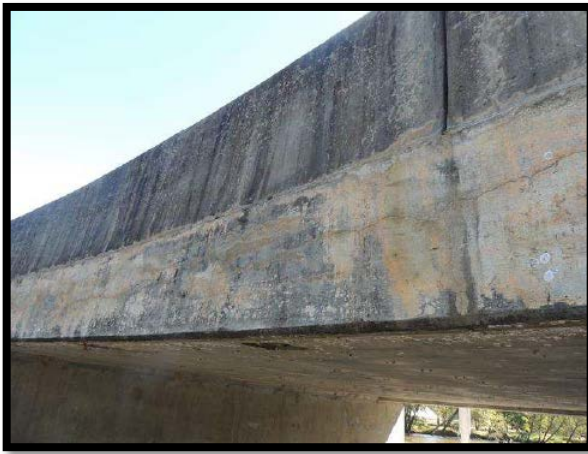
Bridge No. 20 longitudinal cracking of deck, "Indication of structural deterioration"
