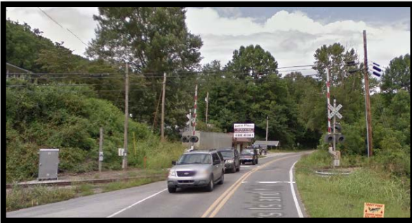
Railroad Crossing on U.S. 19 just east of Bridge No. 20
