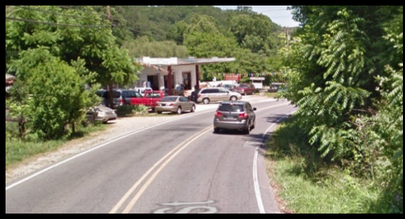
U.S. 19 Headed East, narrow lane width and inadequate shoulders, limited sight distance
