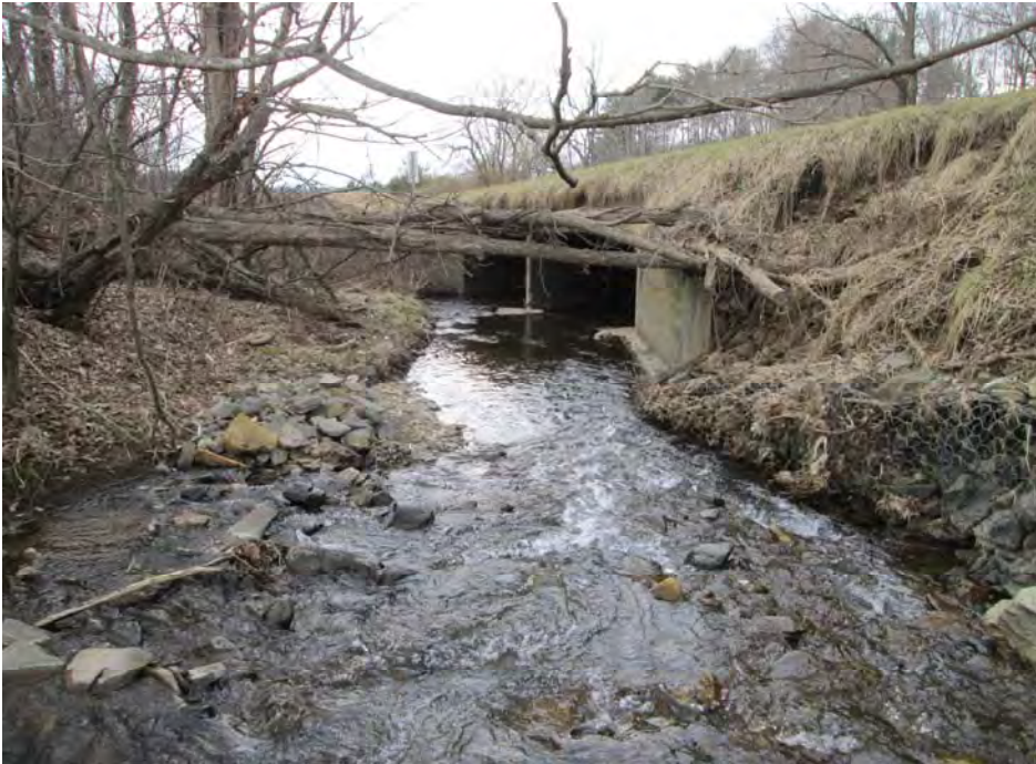
Site 7 – Brushy Fork Creek at US 321 /US 421; upstream face.
