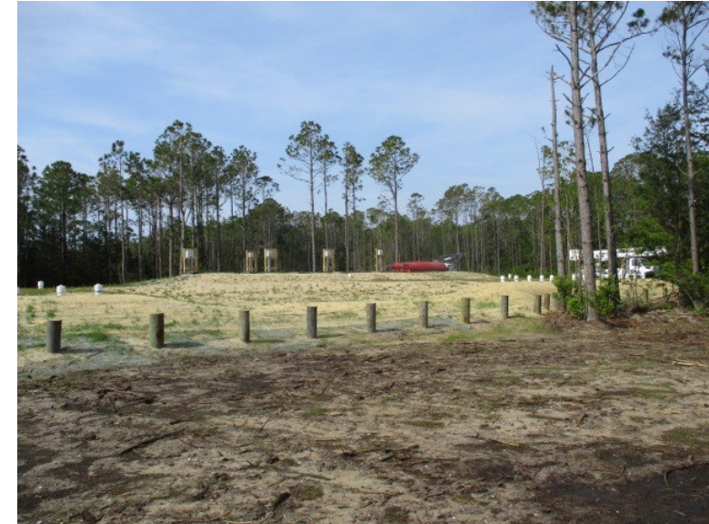
Example of a Drain Field
