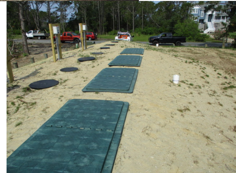
Example of Pre-Treatment Pods for Septic Tanks
