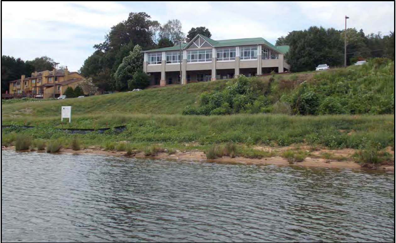
Figure 7. General View of the northern shoreline showing the fill layer, looking north.
