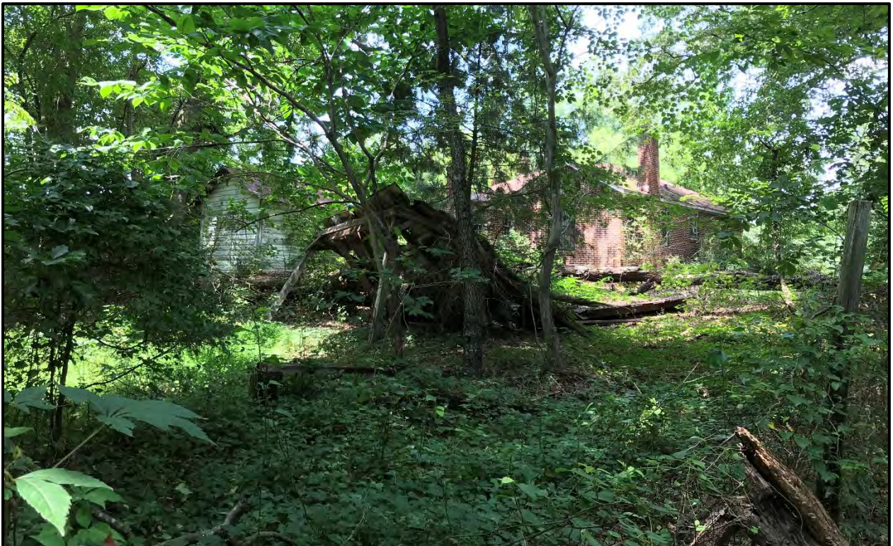
Figure 6. General View of the house at the northwestern end of the parcel west of the US 321 and Alex Lee Road intersection, looking north.
