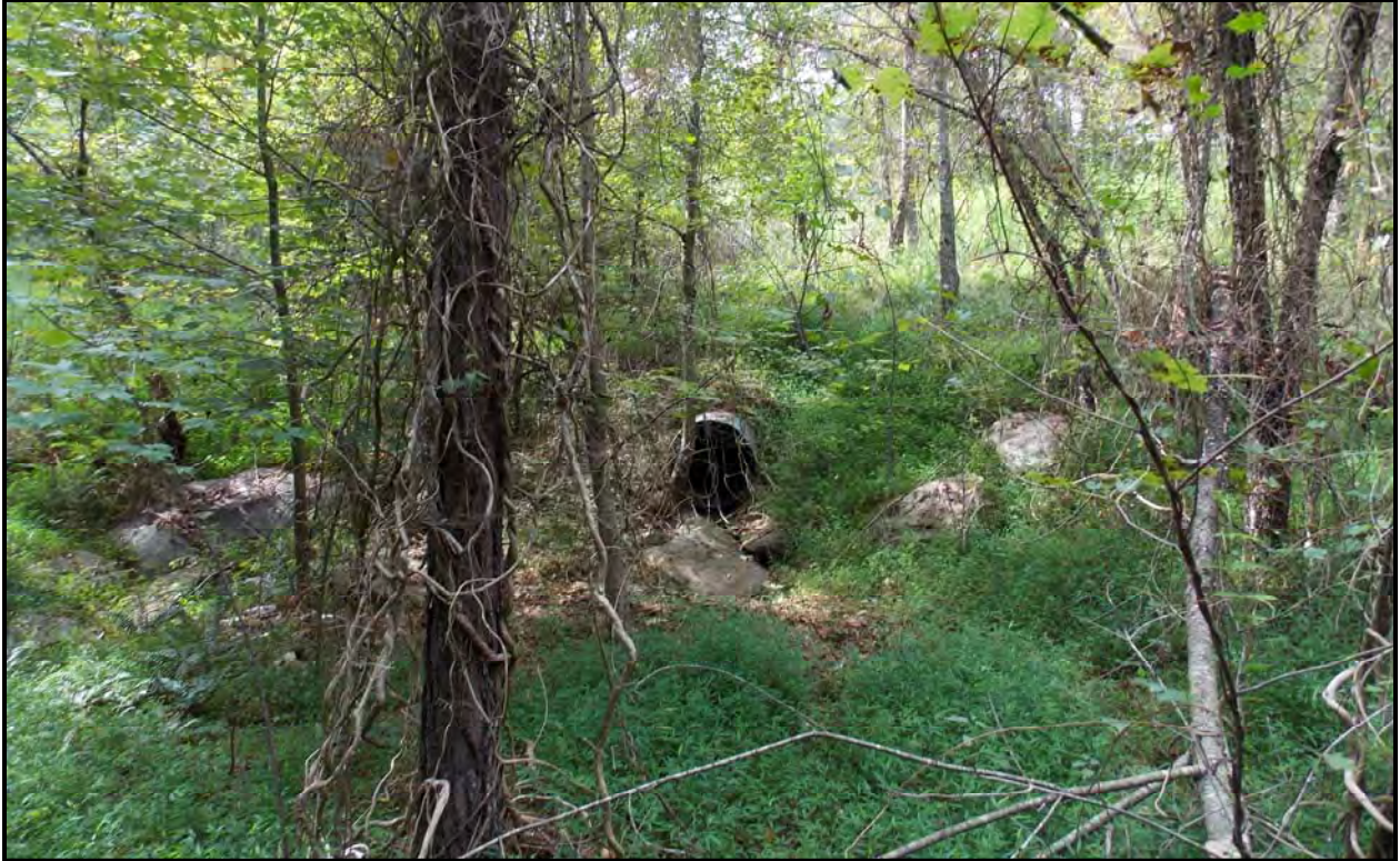
Figure 15. View of the culvert going into the ridge, looking north.
