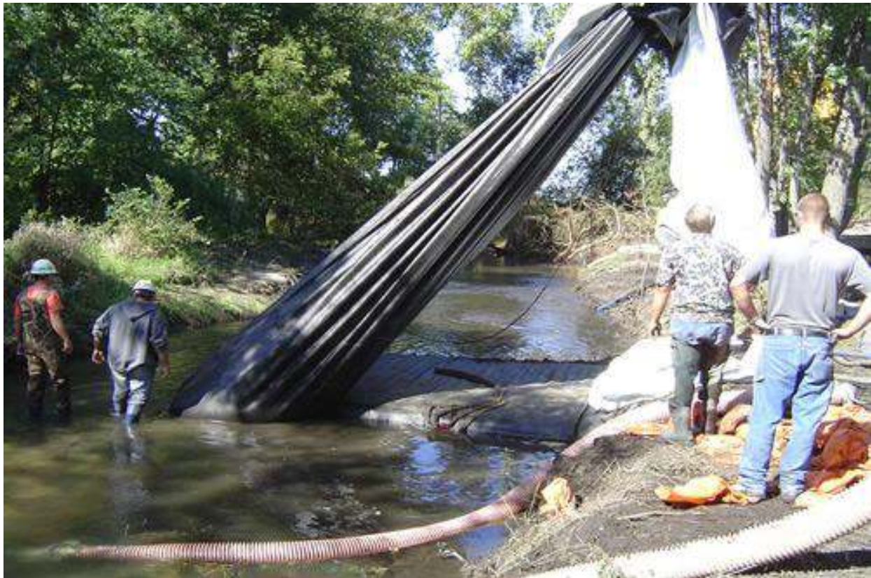
Figure 29 – Workers draining water during removal of a small cofferdam.
