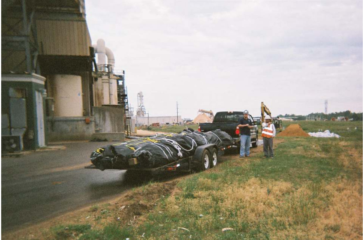
Figure 14 – Rolled up cofferdams arrive on a flatbed at the project site.
