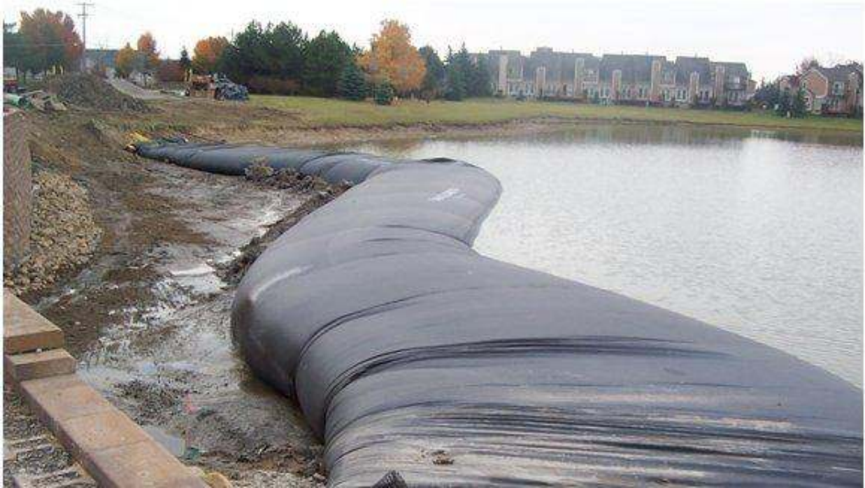
Figure 4 – Dam-It Dams’ cofferdams can withstand tremendous lateral pressure.
