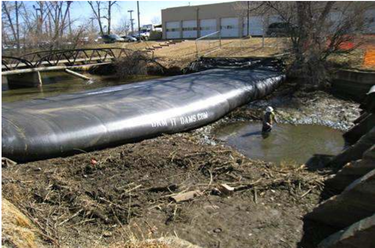
Figure 1 – A fully inflated cofferdam holds back water from the work site.
