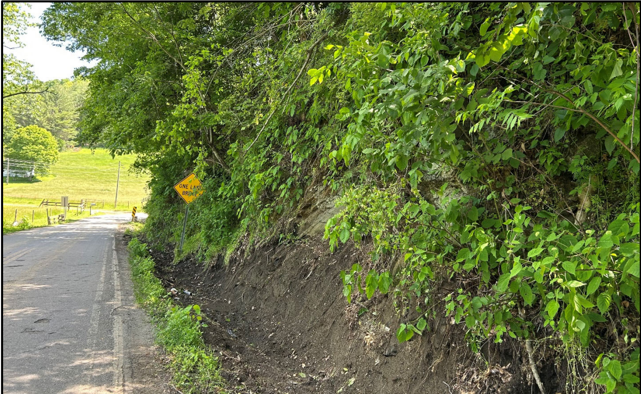
Figure 7. General view of cut hillside in the northwest quadrant, looking south.
