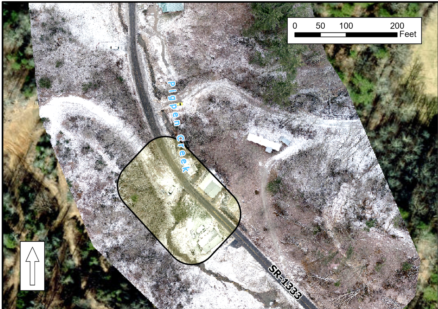
Figure 2. Aerial photography showing the setting for Br. No. 0192 over Pigpen Creek on SR 1333, Upper Pig Pen Road. The image shows conditions after flood damage and emergency repair (January 2025, snowy). The approximate APE is shaded yellow with a black outline.
