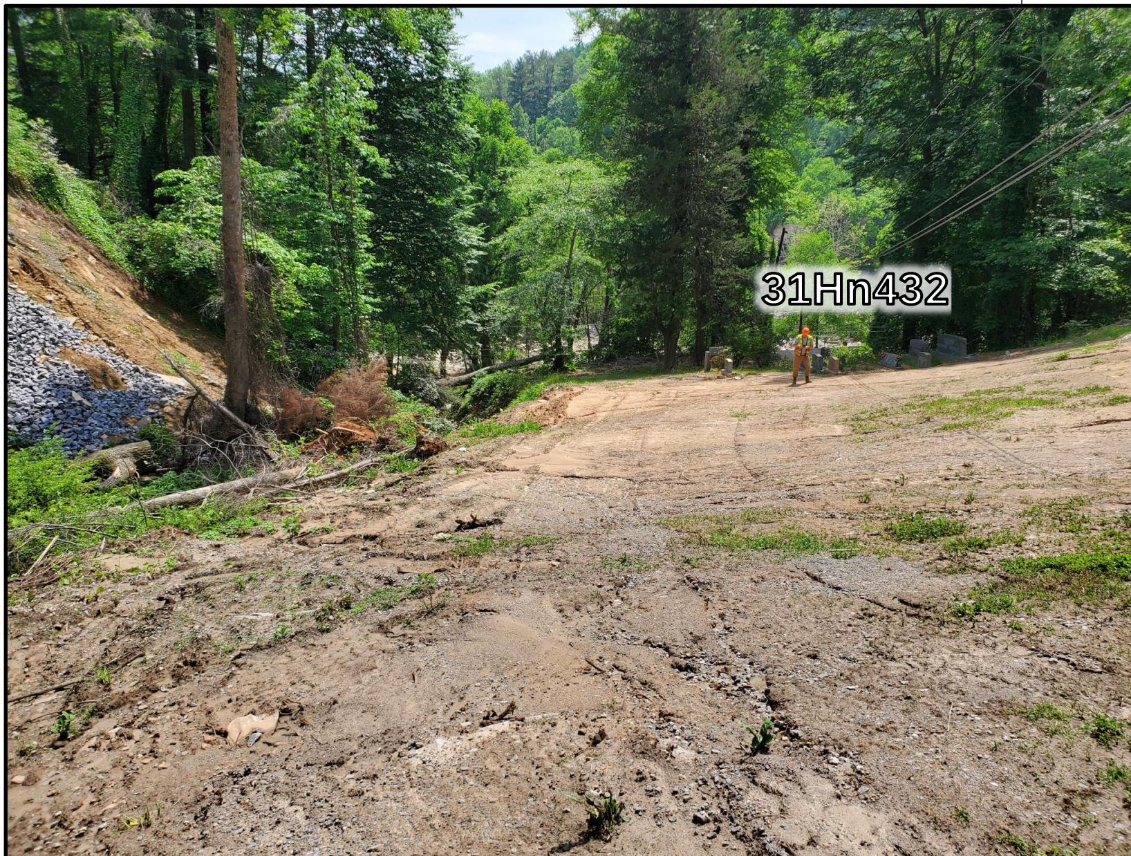
Figure 6. Aftermath of Helene-induced mountain slides above Conner Cemetery, facing southeast. The cemetery is seen in the upper right corner. Possum Hollow Rd. is just beyond the picture frame. Note grading and slope stabilization.
