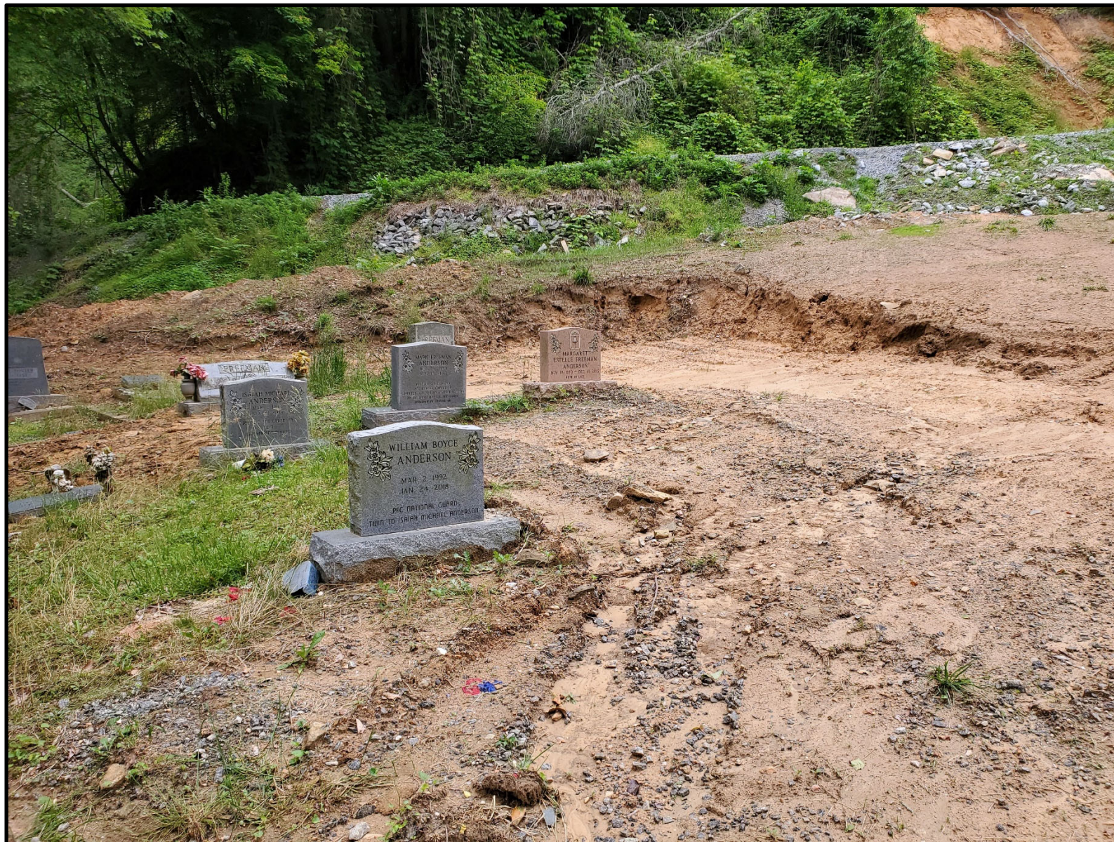
Figure 4. View of Conner Cemetery, facing west on the northern section adjacent to Possom Hollow Road, which has been temporarily repaired following a mountain slide cause by Helene's rains. The photograph highlights that a significant amount of this slide's overburden has been removed from around these northern gravestones.
