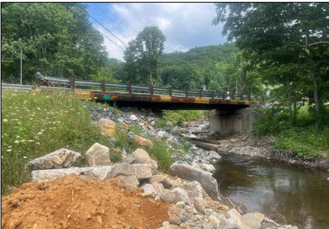
Figure 7: North view of the bridge.
