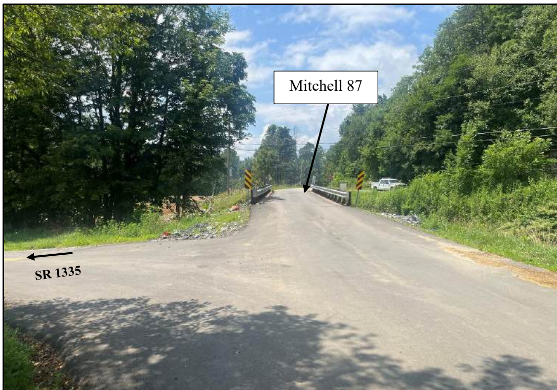
Figure 6: South view of the bridge.
