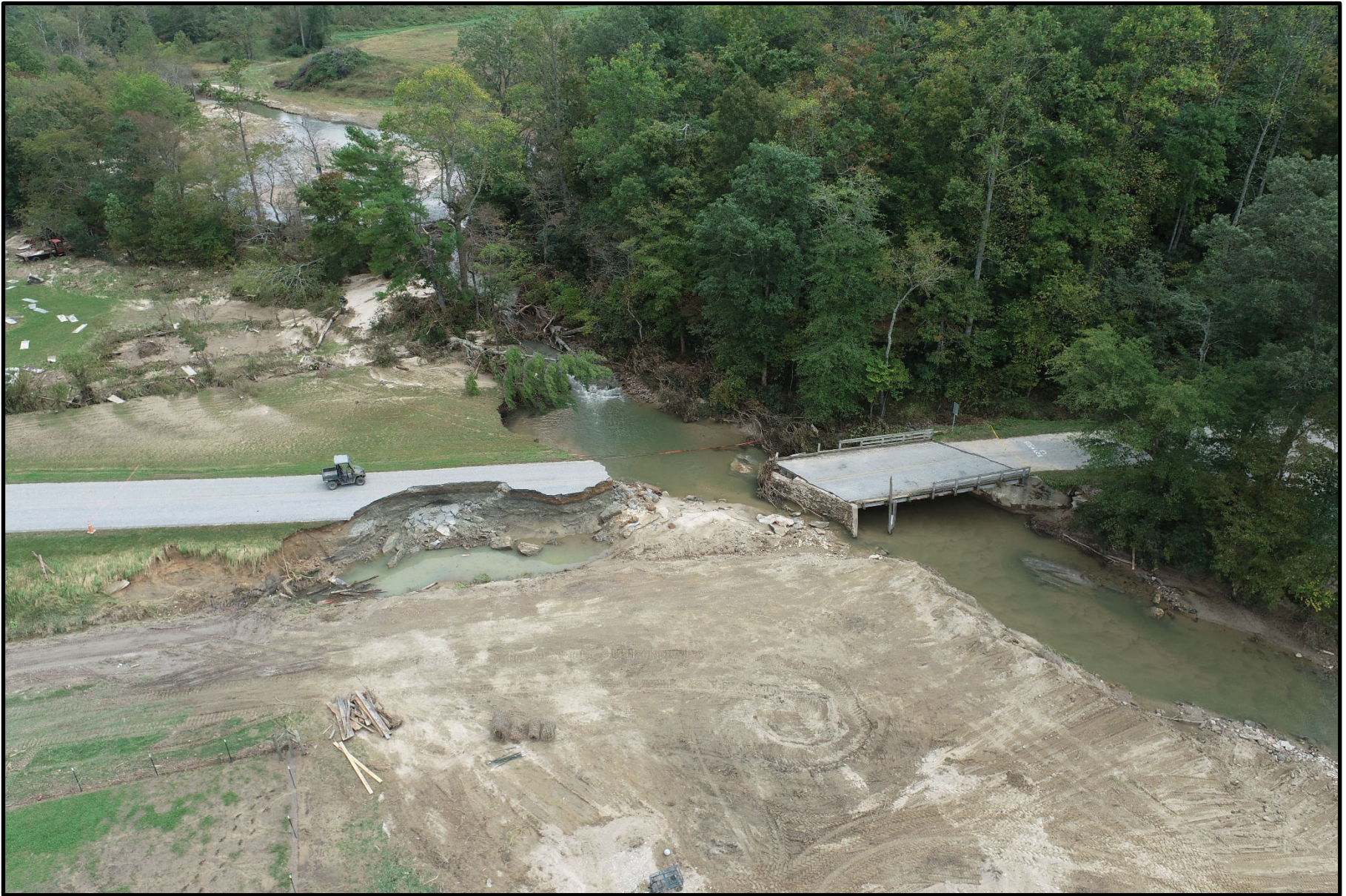
Figure 3. Drone photography of Bridge No. 0198 on SR 1614, Waters Road, showing scouring of the terrain and destruction of the bridge from flooding, facing East (Helene 2024).
