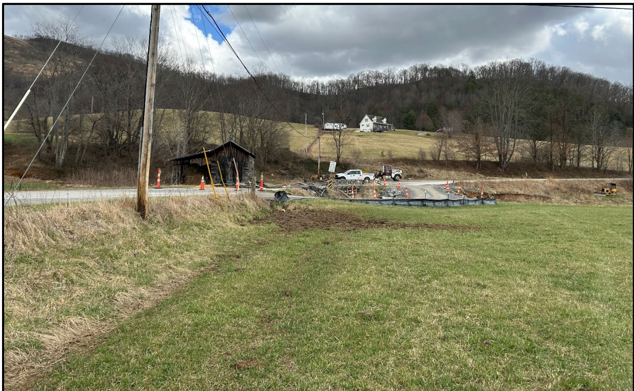
Figure 10. General view of the southwest quadrant, looking east.
