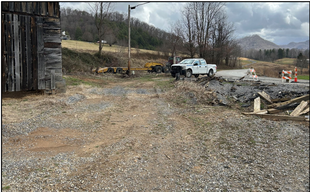
Figure 8. General view of the northeast quadrant showing gravel layer after cleanup of debris, looking southeast.
