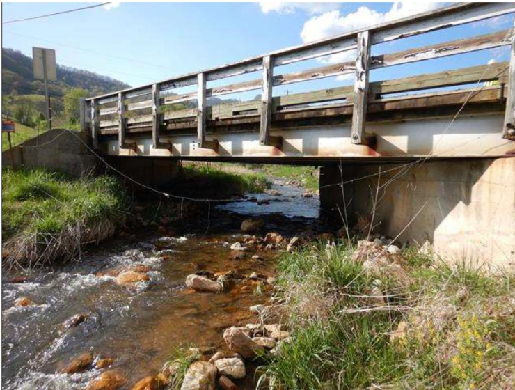
DOWNSTREAM PROFILE, LOOKING EAST
