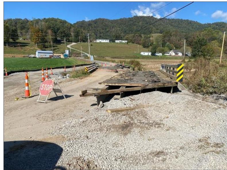
south approach looking north
