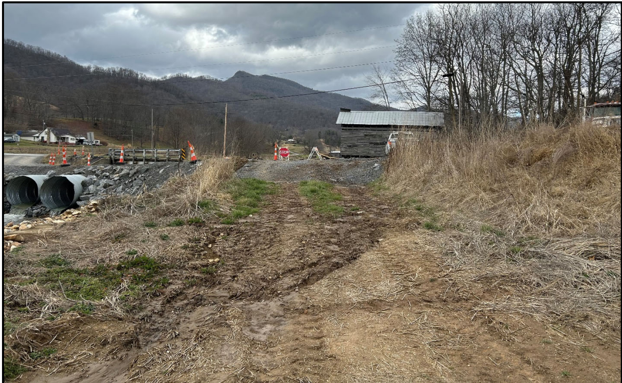
Figure 9. General view of fill for the access drive in the southeast quadrant, looking north.
