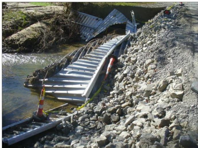
PAR: CULVERT FOLDED UNDER ON UPSTREAM END
