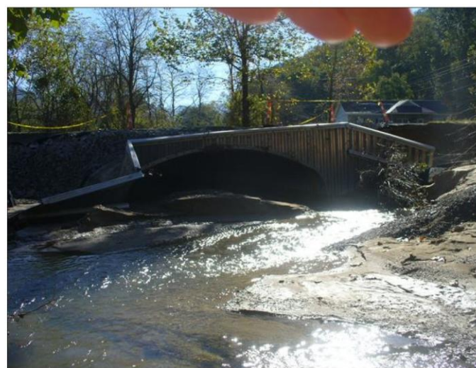
PAR: DAMAGED WEST SIDE HEADWALL
