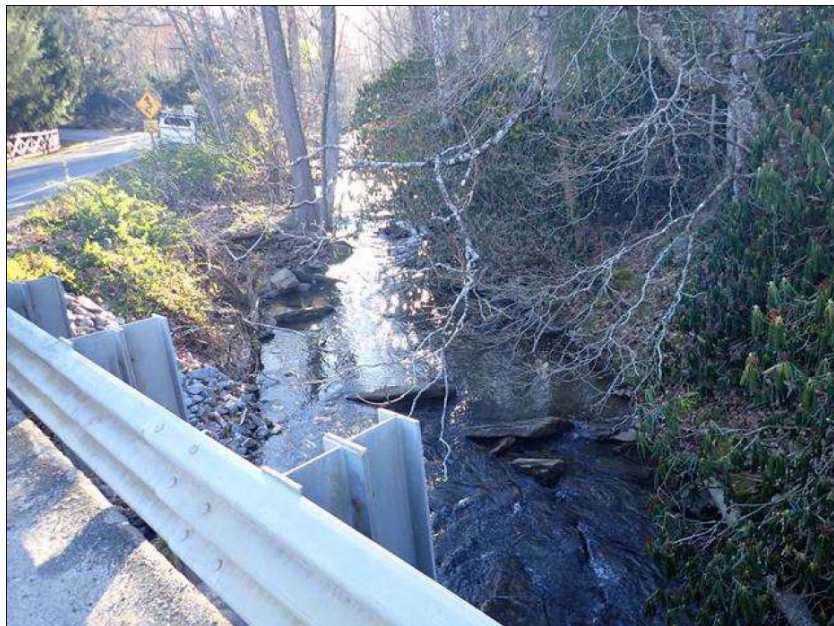
looking upstream from deck (east)
