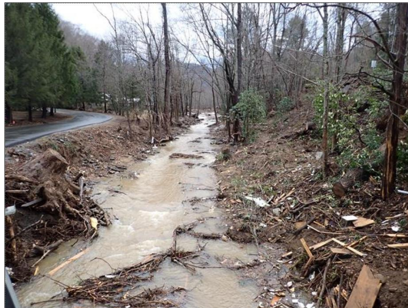
LOOKING EAST FROM STRUCTURE (UPSTREAM)
