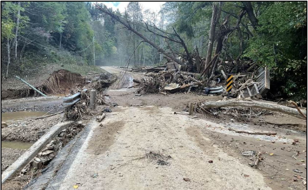
Figure 3. Hurricane Helene damage to Bridge No. 424 and landforms along Flat Creek Road.
