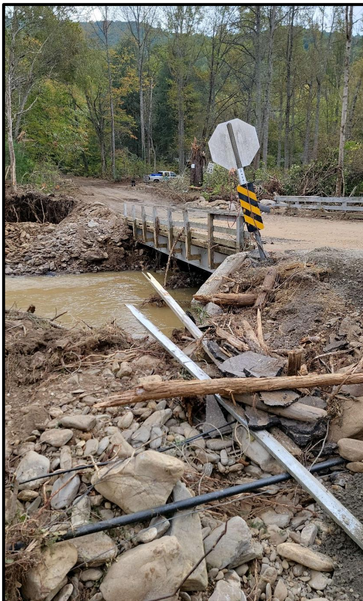
Figure 6: General Photo of Project Area Conditions post Hurricane Helene, dated 10 Oct 2024 (from NCDOT Hurricane Helene All Imagery/Drone Map).
