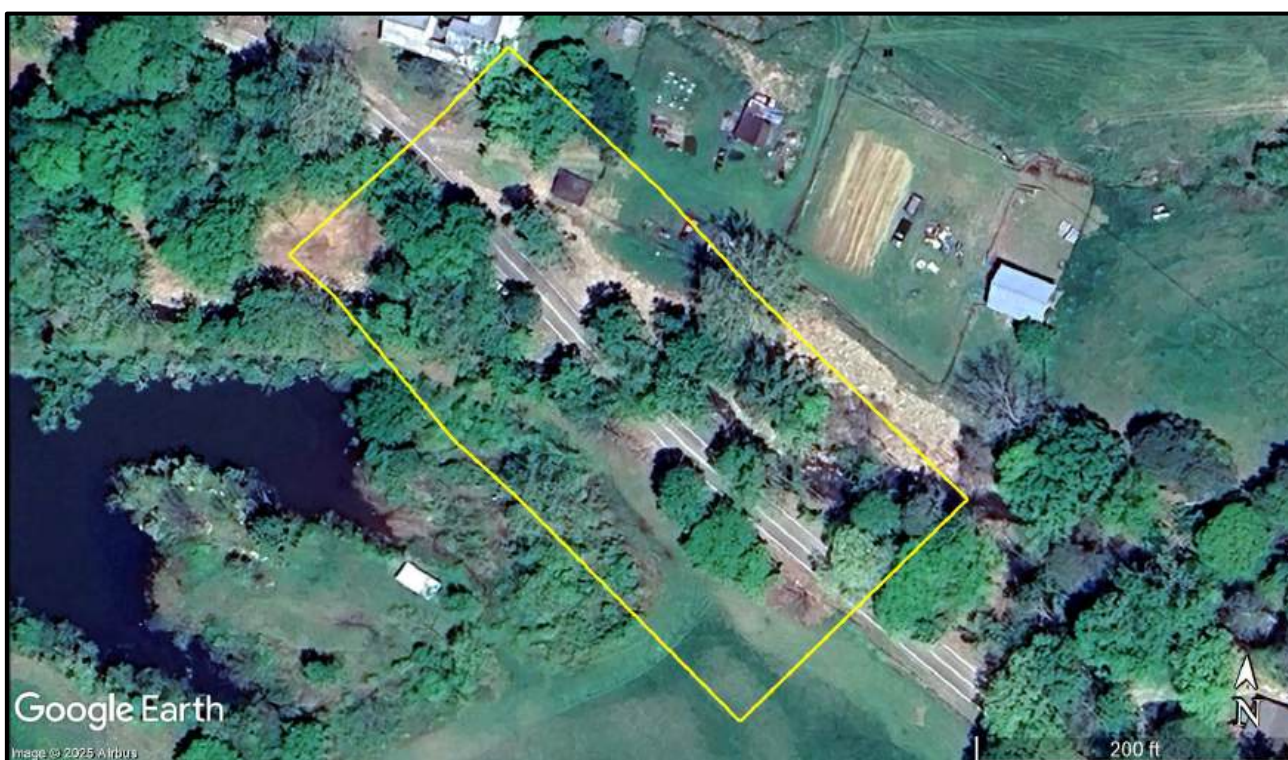
Figure 6. Google Earth Imagery from April 28, 2025, showing scouring of floodplain after Hurricane Helene northeast, northwest and southeast of Bridge 159. Project APE is depicted in yellow.
