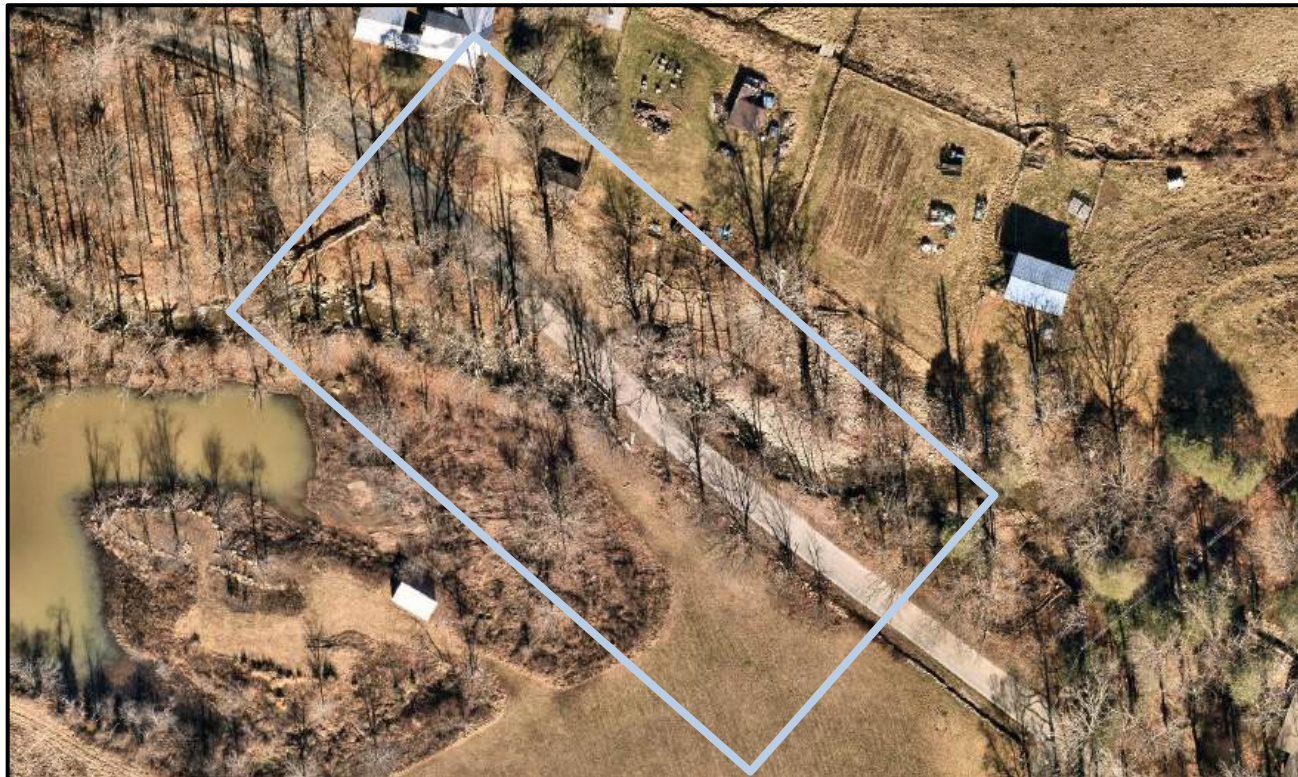
Figure 7. Nearmap Imagery from January 28, 2025, showing scouring of floodplain after Hurricane Helene northeast, northwest and southeast of Bridge 159. Project APE is depicted in light blue.
