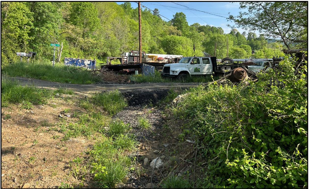
Figure 9. View of the northeast quadrant showing soil erosion from flooding, looking north.
