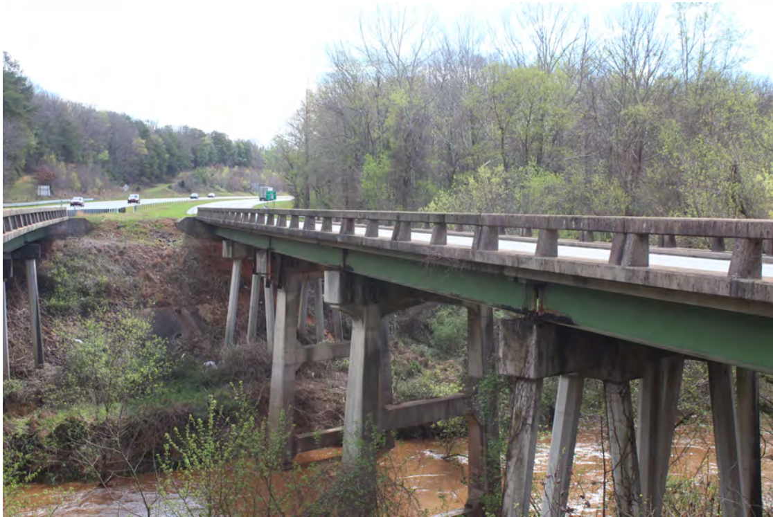
North face of Bridge 83 (US 74 Bypass East)
