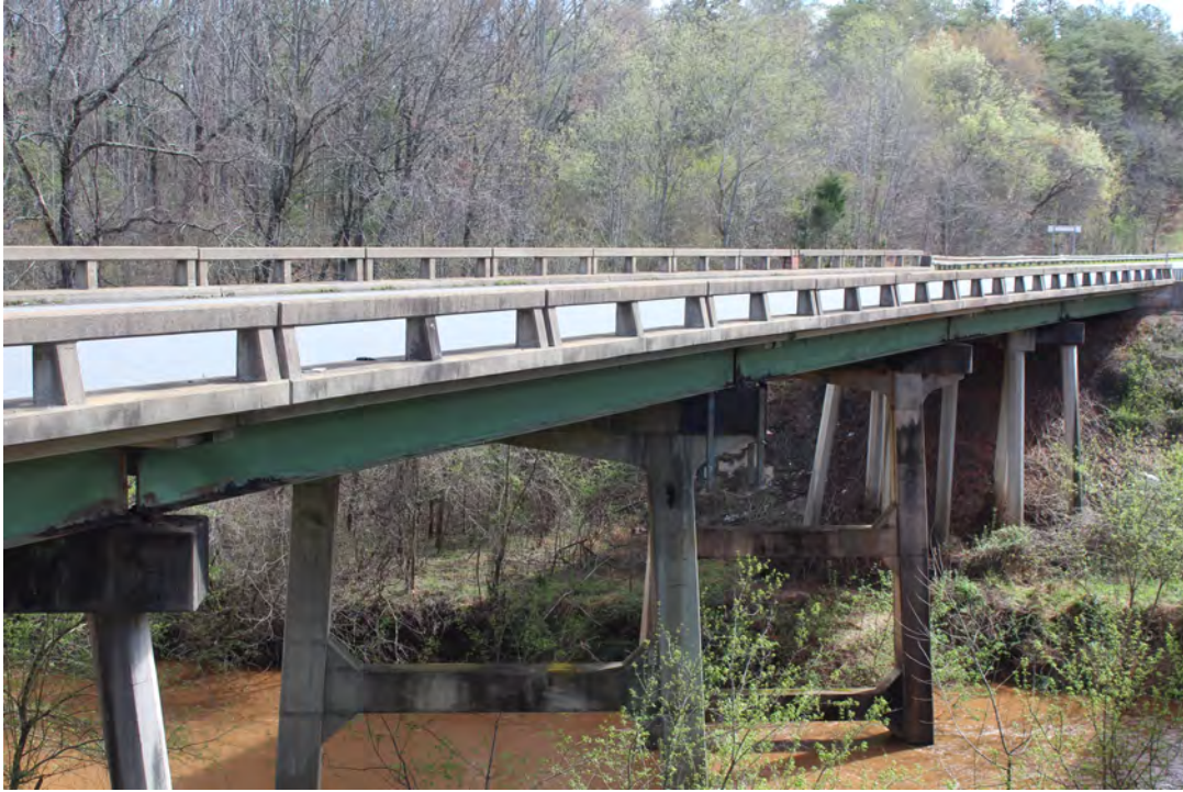
South face of Bridge 84 (US 74 Bypass West)
