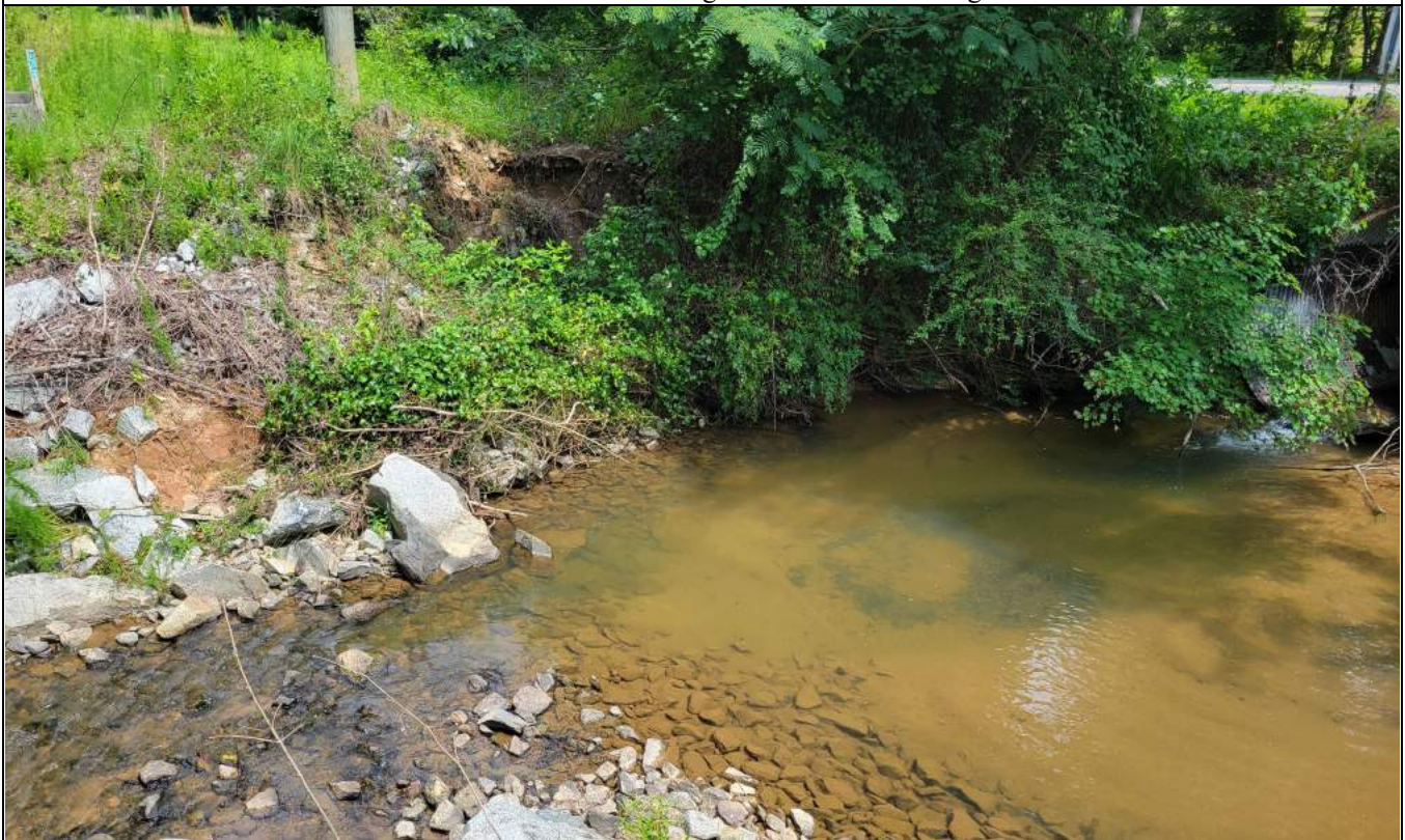
Photo 2 – This photo depicts the view slightly further downstream of the existing culvert outlet carrying Kerners Mill Creek under Hopkins Road at Impact Site 4A. Note the large scour hole at the base of the culvert outlet.
