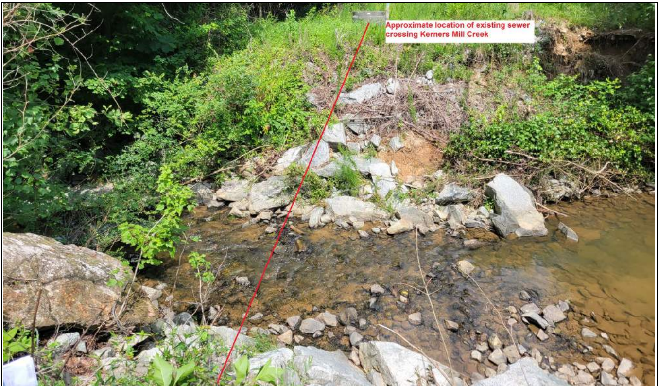
Photo 3 – This photo depicts the view of the existing sewer crossing below Kerners Mill Creek at Impact Site 4A. The proposed 12-inch sewer line realignment will be installed within in a 20-inch steel encasement pipe fastened to subgrade concrete support piers located outside on either side of the stream to provide additional stabilization.
