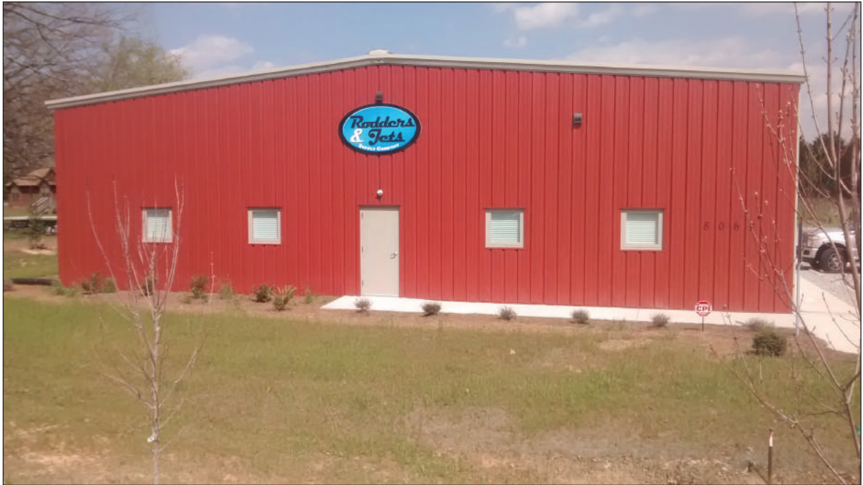
Figure 15. View of Survey Area 6
