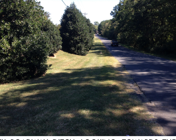
EX ROADWAY DITCH LOOKING TOWARDS THE 18" CMP CROSSPIPE INLET
