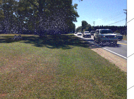
EX SWALE ON HISTORIC PROPERTY
