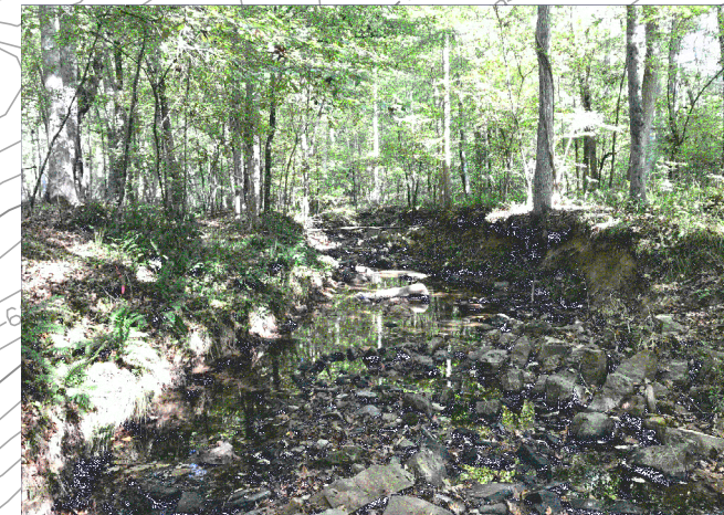
MUNDY'S RUN CREEK DOWNSTREAM OF CULVERT SITE LOOKING UPSTREAM.
