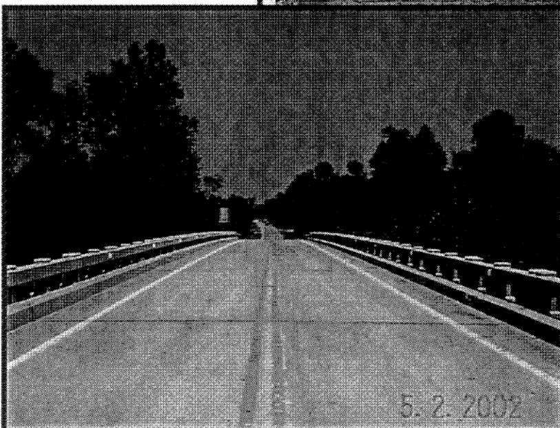
View of west approach from Bridge No. 21
