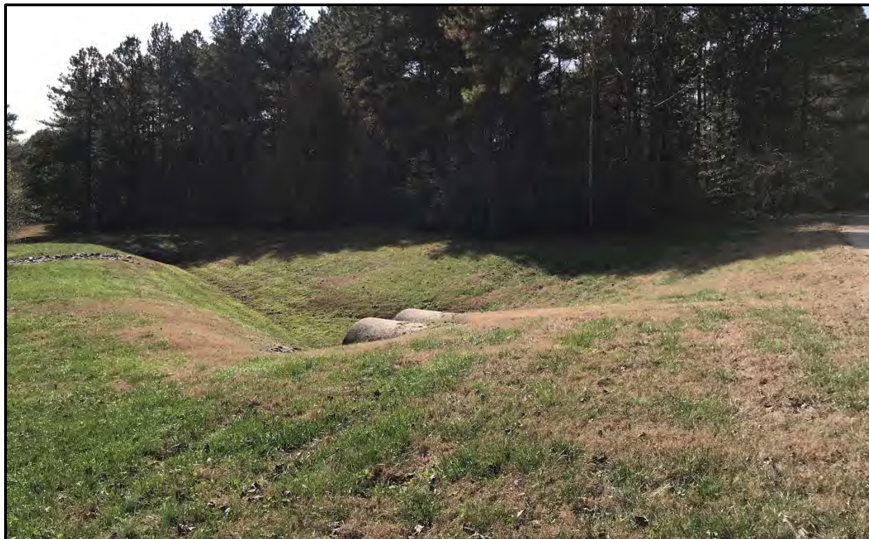
Figure 3. General View of storm drainage ditch disturbance within the APE, looking southwest.
