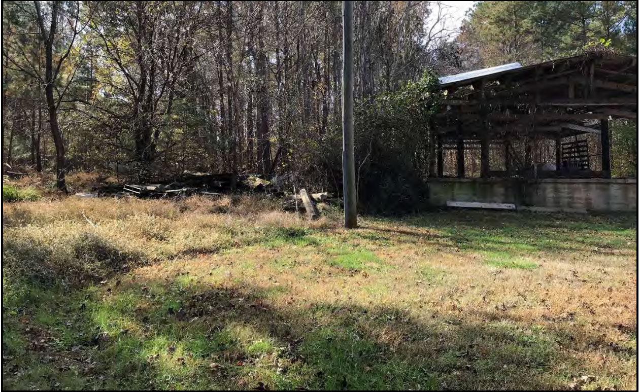
Figure 5. General View south of the Sports Endeavors complex showing push pile and shed, looking east.
