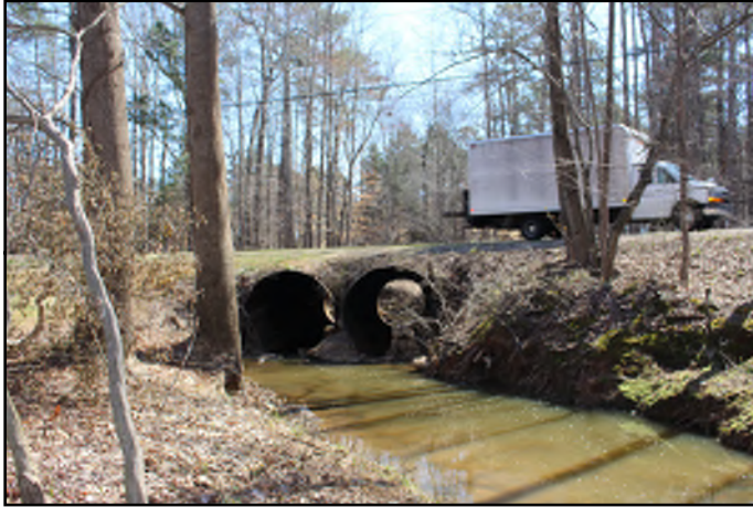
Culverts carrying Williams Creek under Lake Pine Drive
