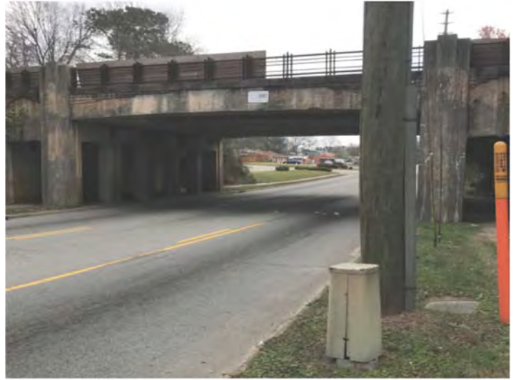
Existing CSX Railroad Bridge
