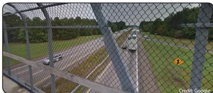
Existing view from pedestrian bridge west toward Wade Avenue
