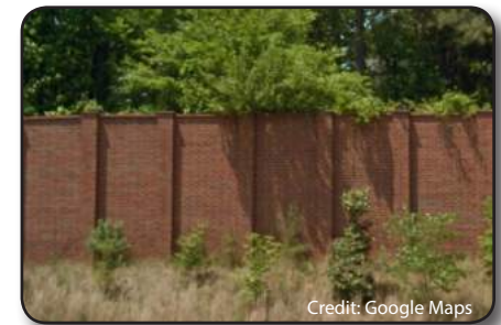
Existing noise wall along I-440 west of Lake Boone Trail
