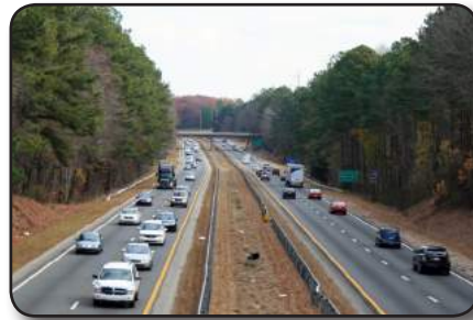
Typical I-440 in the project area
