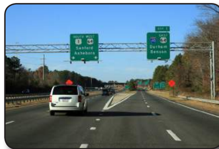
Collector-Distributor road to I-40 ramps
