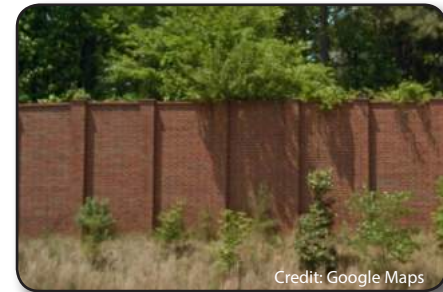
Existing noise wall along I-440 west of Lake Boone Trail
