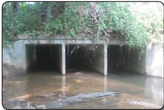
The outlet of the Walnut Creek triple-box culvert under I-440.
