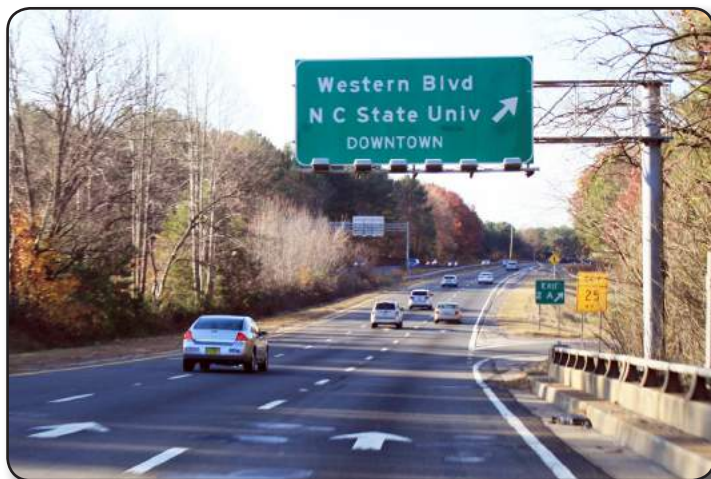
Example: No deceleration lane and inadequate shoulder at Western Boulevard exit
