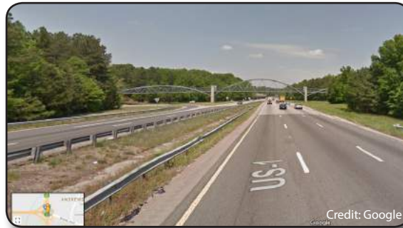
Existing view from I-440 north to pedestrian bridge
