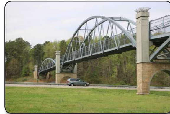
Reedy Creek Greenway pedestrian bridge over I-440
