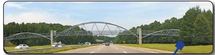
Reedy Creek Trail pedestrian bridge over I-440 north of Wade Avenue
