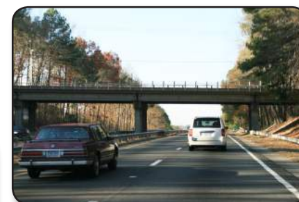
Athens Drive bridge - rated structurally deficient
