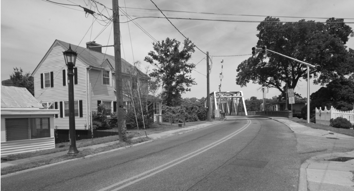
Figure II-3 Existing US 17 Business/NC 37 south of Bridge Number 8 in Hertford (looking north)
