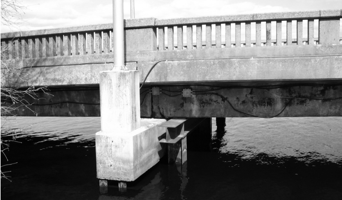
Figure II-2 Steel crutch bents under existing bridge
