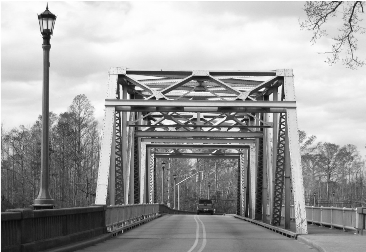
Figure II-4 Existing US 17 Business/NC 37 on Bridge Number 8 (looking north)
