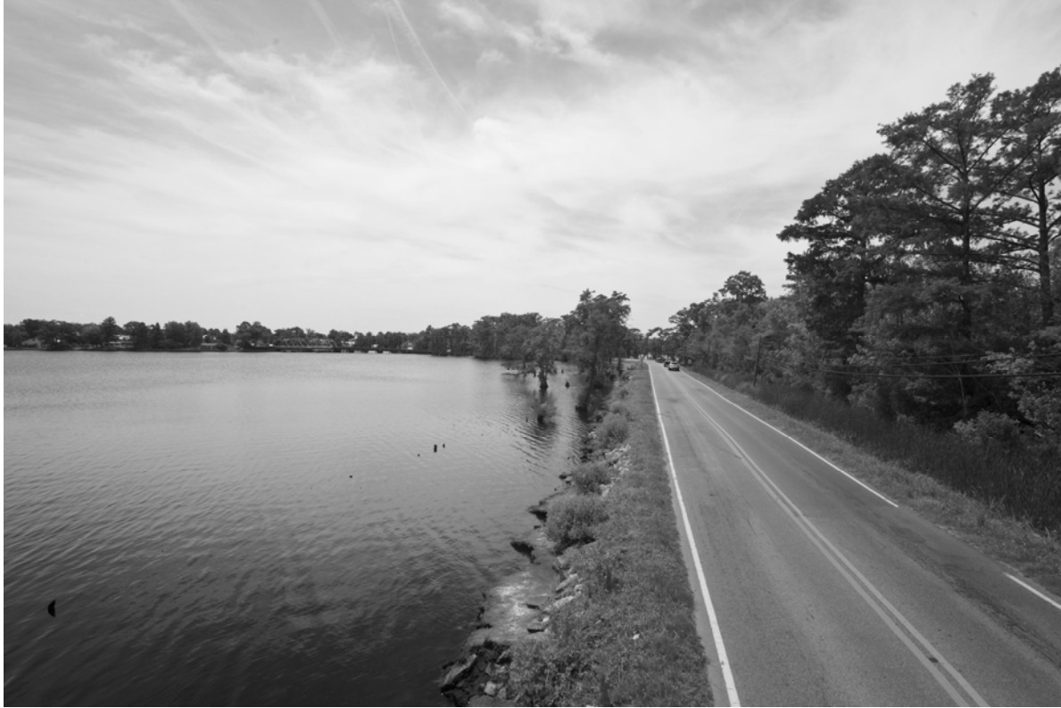
Figure II-5 Existing US 17 Business/NC 37 on the causeway north of Bridge Number 8 (looking south)
