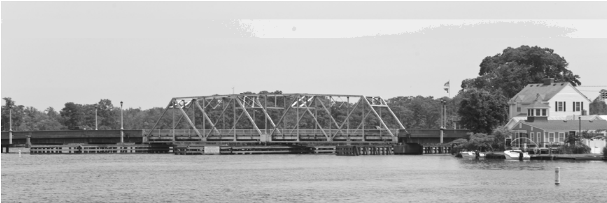
Figure II-6 Existing Bridge Number 8 (looking east)
