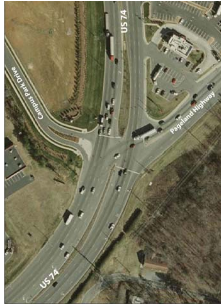
Figure 7 – Intersection of US 74 and Pageland Highway U.S. Department of the Interior U.S. Geological Survey, 2007
