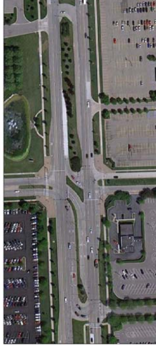
Figure 5 – Superstreet intersection of W. Big Beaver Rd. and Lakeview Dr., Troy, MI Imagery ©2013 DigitalGlobe, GeoEye, U.S. Geological Survey, USDA Farm Service Agency, Map Data ©2013 Google
