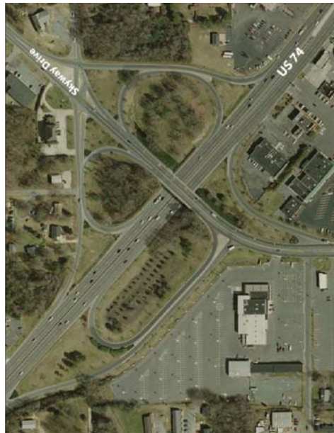
Figure 8 – Intersection of Skyway Dr. and US 74, Monroe, NC
