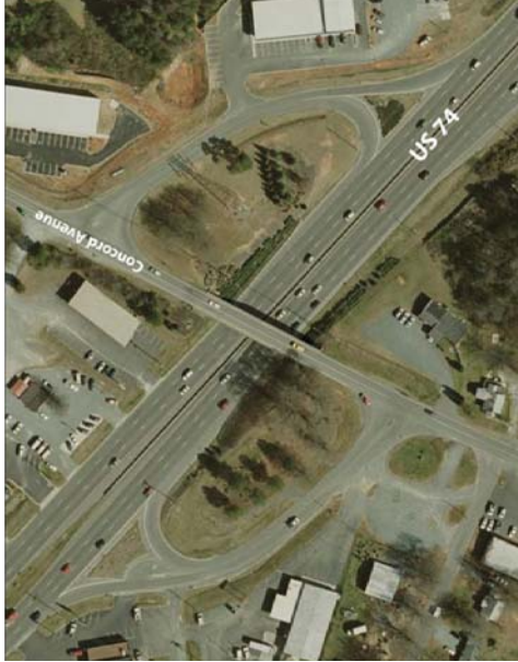
Figure 9 – Intersection of Concord Ave. and US 74, Monroe, NC
