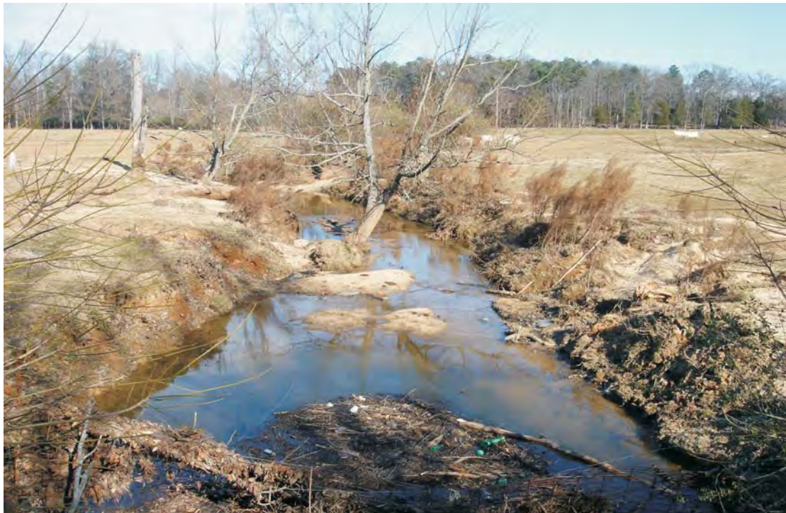
Photo 2: View of eroding banks and extensive sediment deposition within Site 1.
