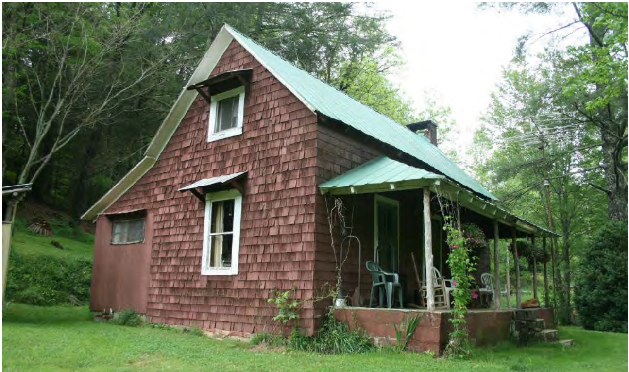
Chapman House, southwest elevation, view to northeast
