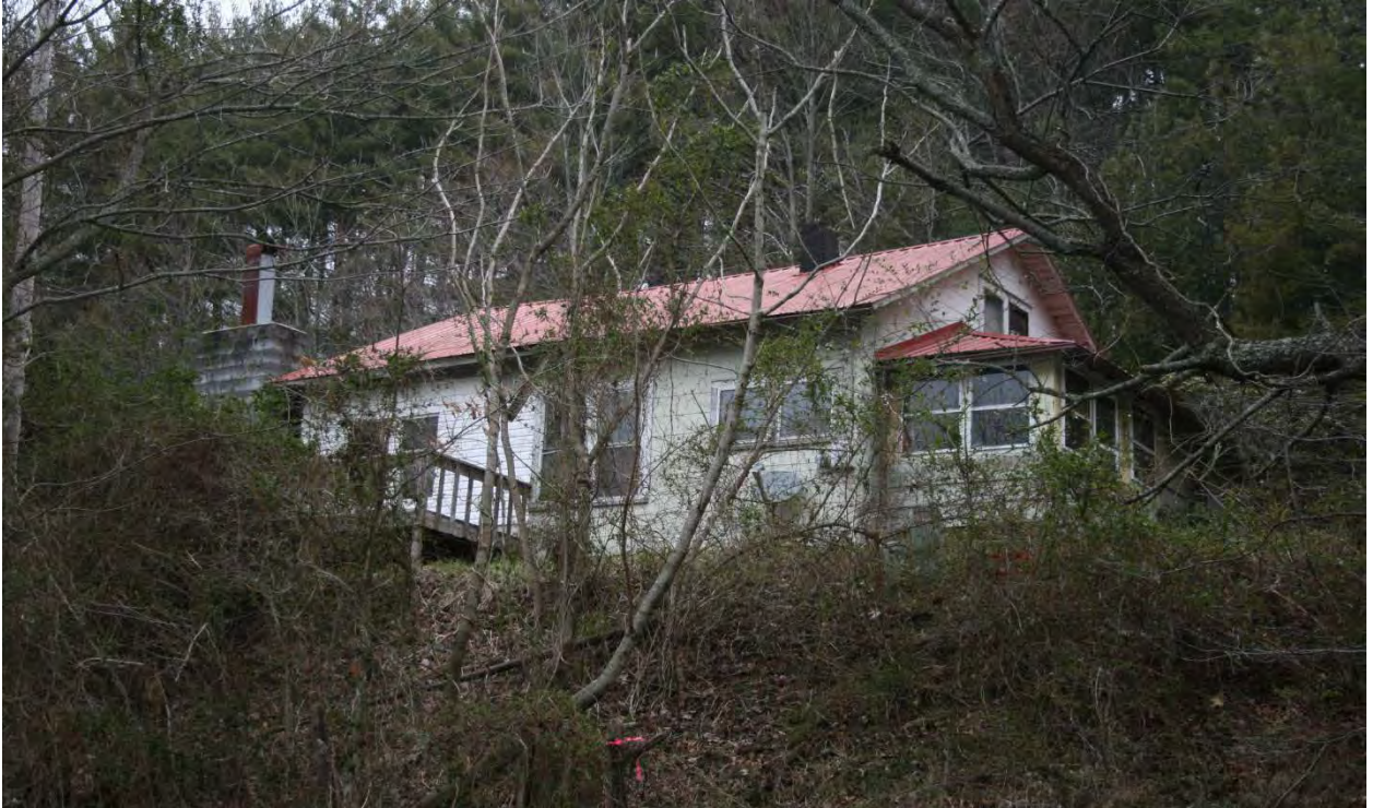
1. House, 107 Reno Drive [PIN 8532-74-3886-000], view to northwest from US 64
