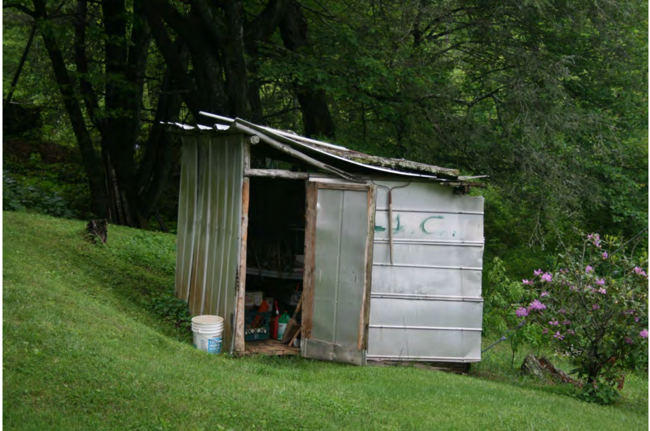
Shed, front view to north
