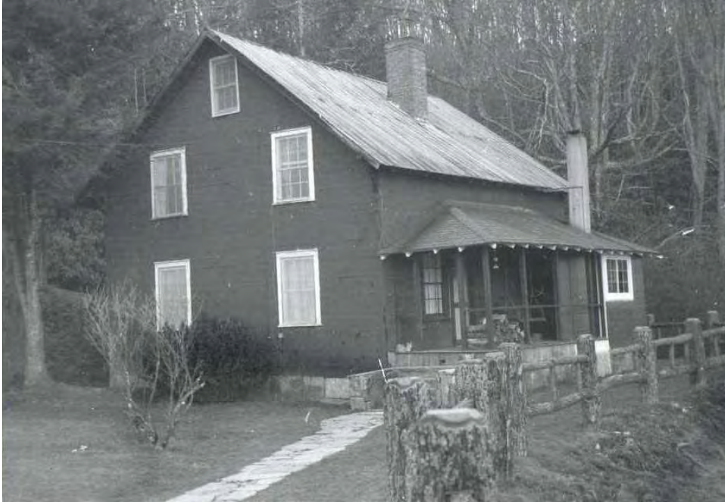
Jason McCall Farm (TV 161), Golden Road (SR 1313) [PIN 8533-71-1024-000], farm house (February 1991), view to northwest
