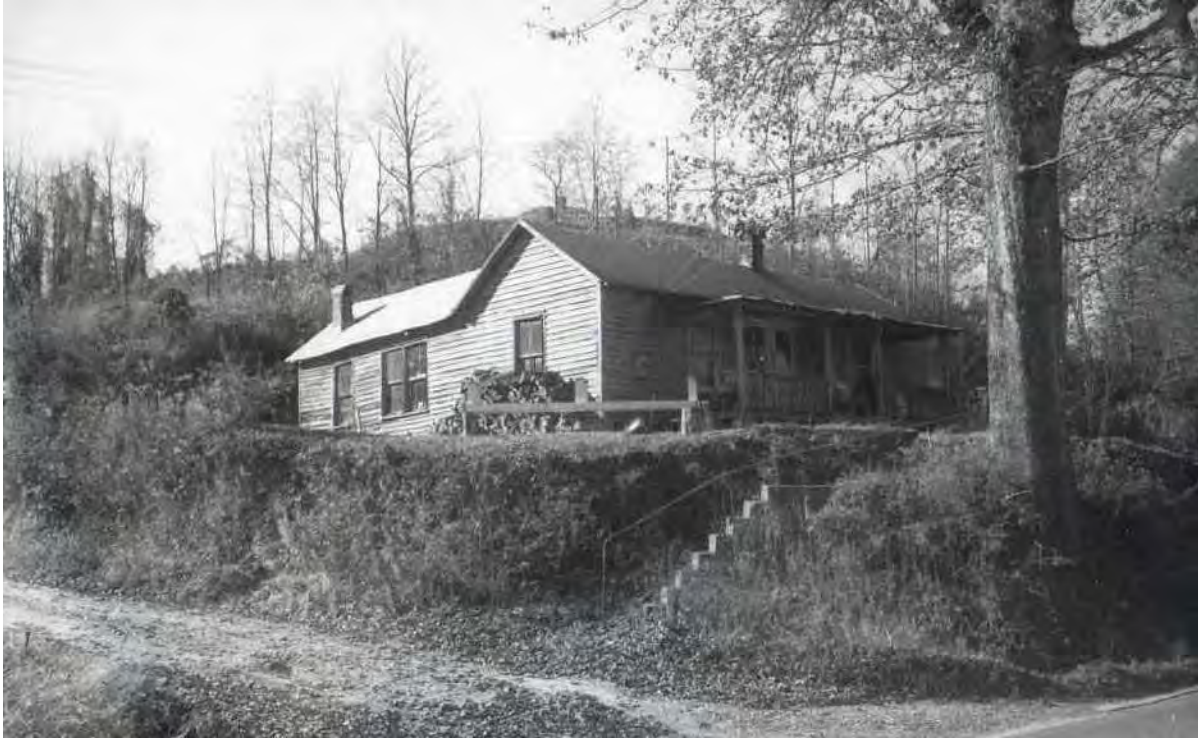
Jordan & Corrine Whitmire Rental House (TV 56), W side of Pickens Hwy (US 178) [PIN 8552-77-3179-000], view to northwest (November 1990)
