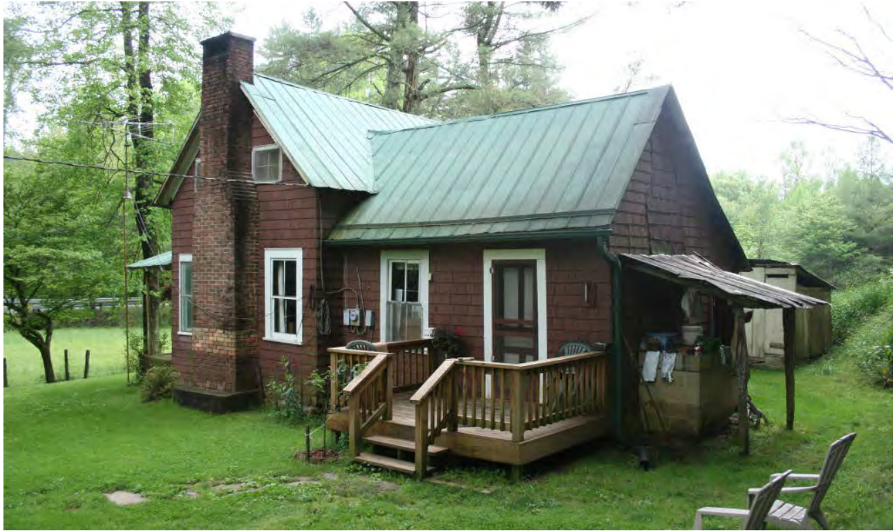
Chapman House, northeast elevation, view to southwest
