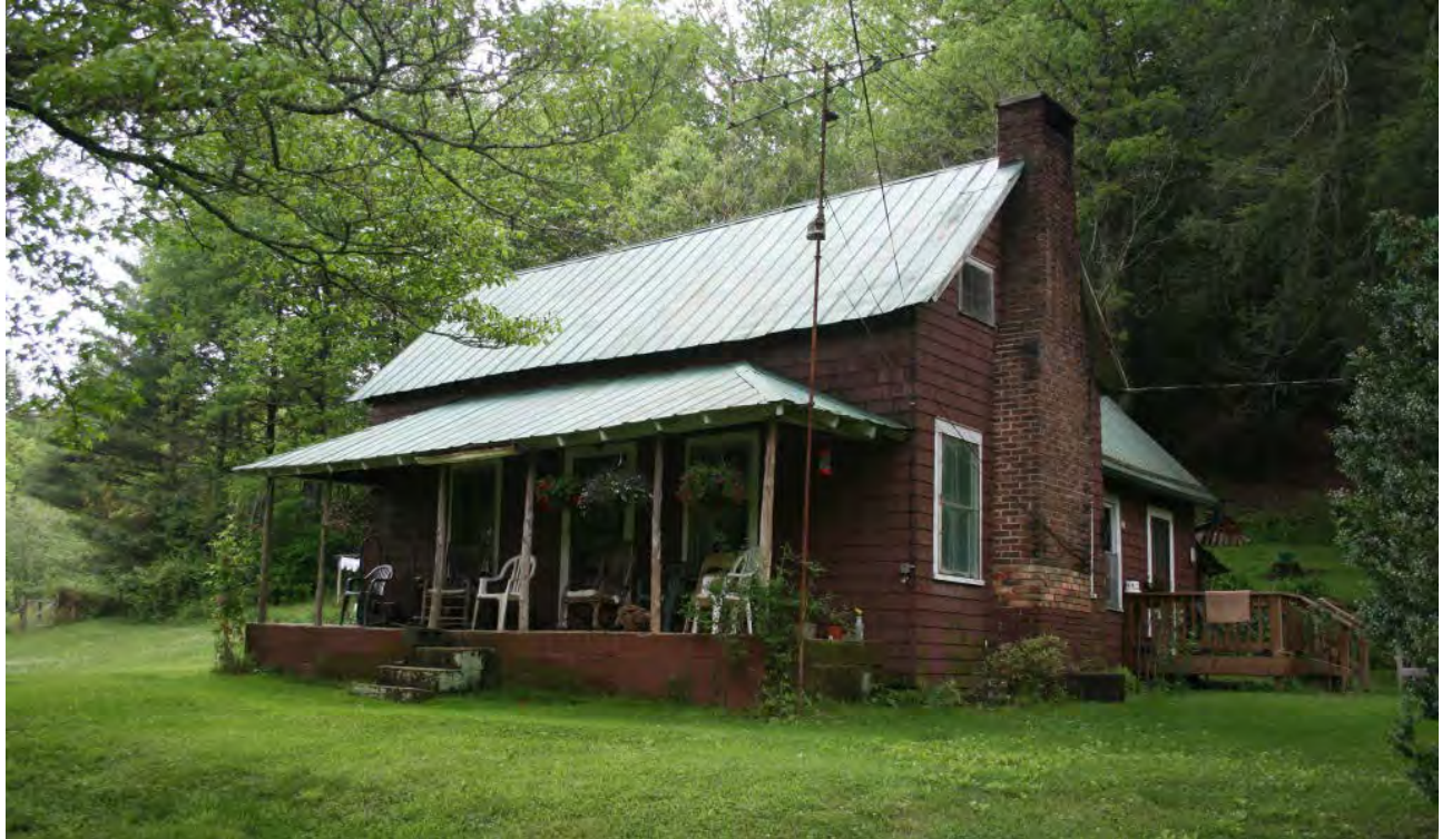
Chapman House, oblique front view to northwest
