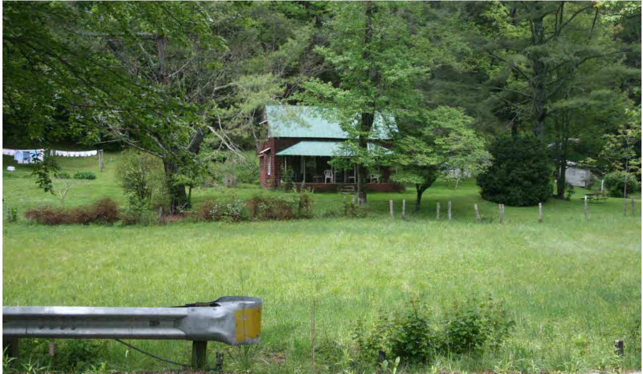
Chapman House, overall view to northwest from US 64 (Rosman Highway)
