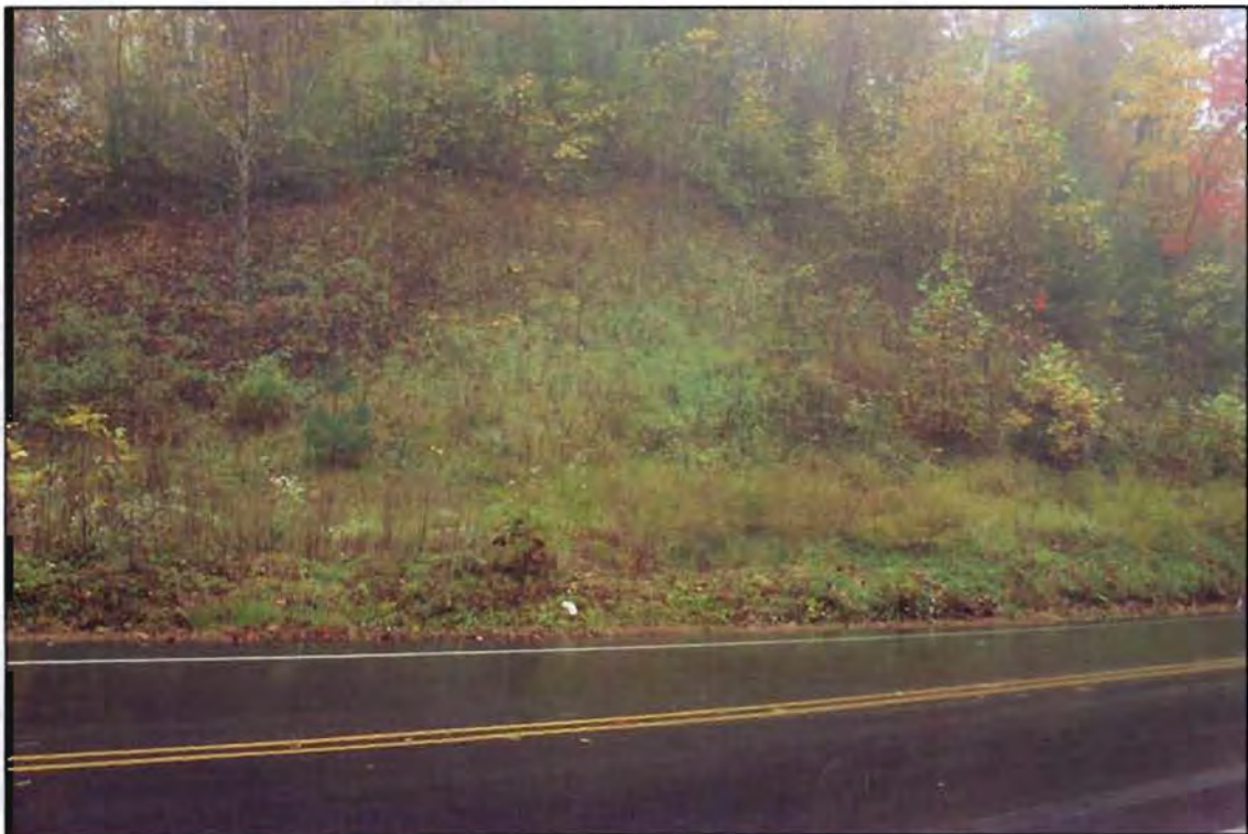
Figure 6. Cut bank along southwest side of APE, view to south.
