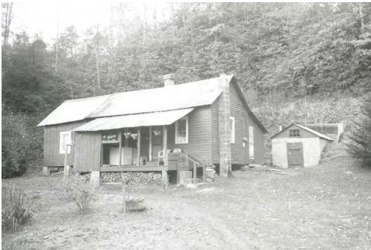
Robby McCall House (TV 19), Old CCC Camp Road (SR 1377) [PIN 8546-33-0190-000], view to west (November 1990)
