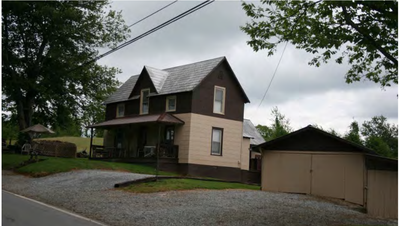
O.L. Erwin House (TV 73), 1054 Catheys Creek Church Road [PIN 8563-14-7031-000], view to east (May 2012)
