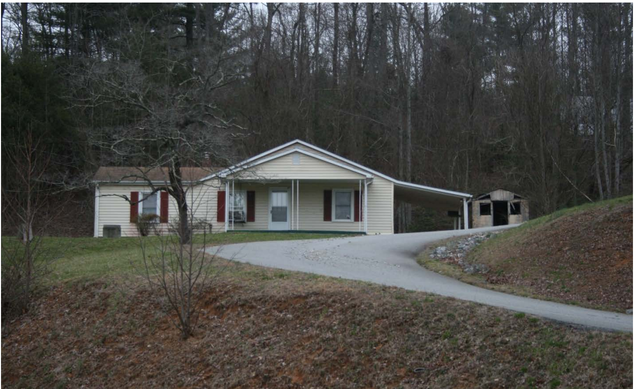
2. House, 39 Carefree Lane [PIN 8532-64-7964-000], view to northeast
