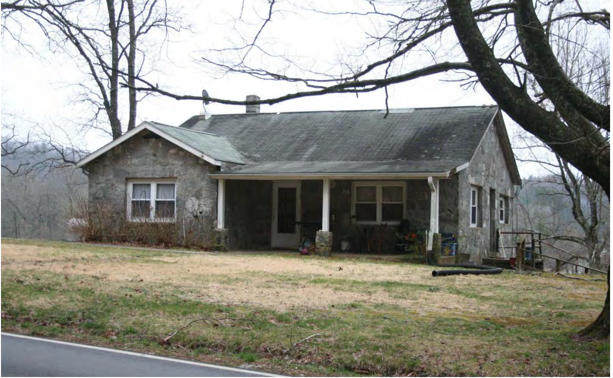
3. House, 12131 Rosman Hwy. [PIN 8532-64-7469-000], view to southeast from US 64
