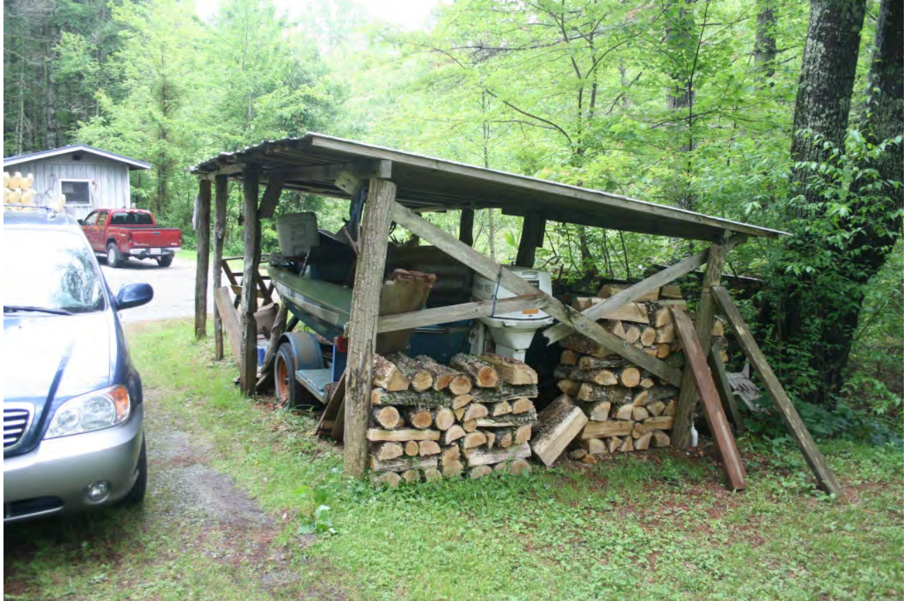
Shed, oblique side view to the northeast
