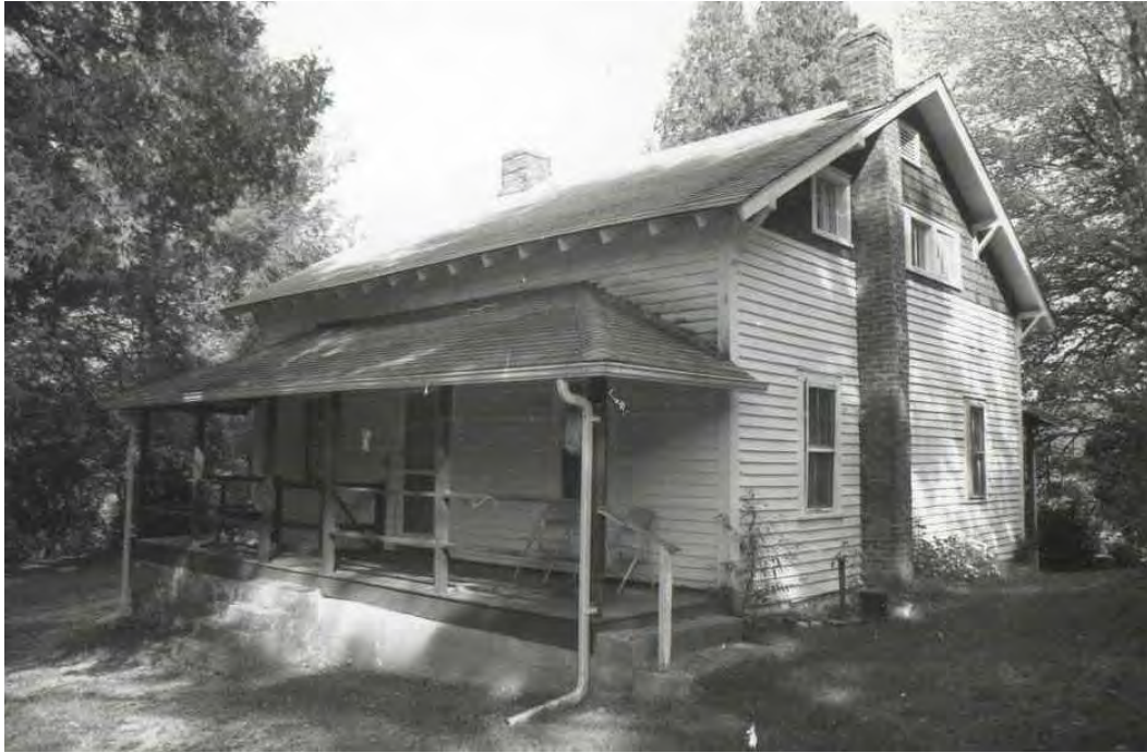
John & Mamie Reid House (TV 500), N side of Old Quebec Road (SR 1318) [PIN 8532-98-5059-000], view to northeast (September 1991)
