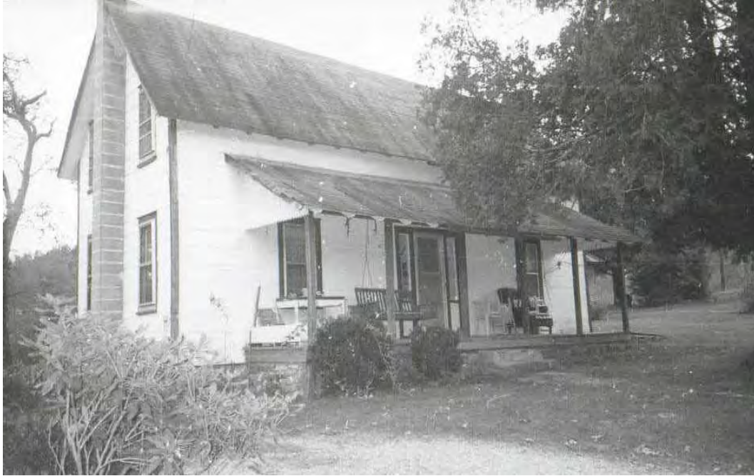
Rufus & Elvira McCall House (TV 10), W side of Shoal Creek Road (SR 1327) [PIN 8546-75-7216-000], view to southwest (November 1990)
