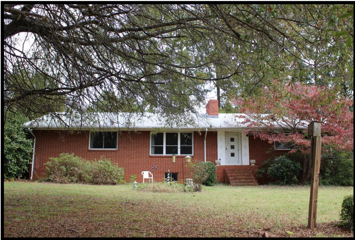
Figure 15: Chester Farmstead, Ranch Dwelling, Looking East.
