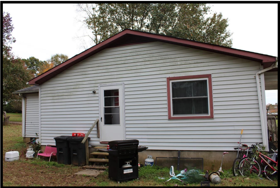
Figure 11: Chester Farmstead, Second Dwelling, Looking Southeast.
