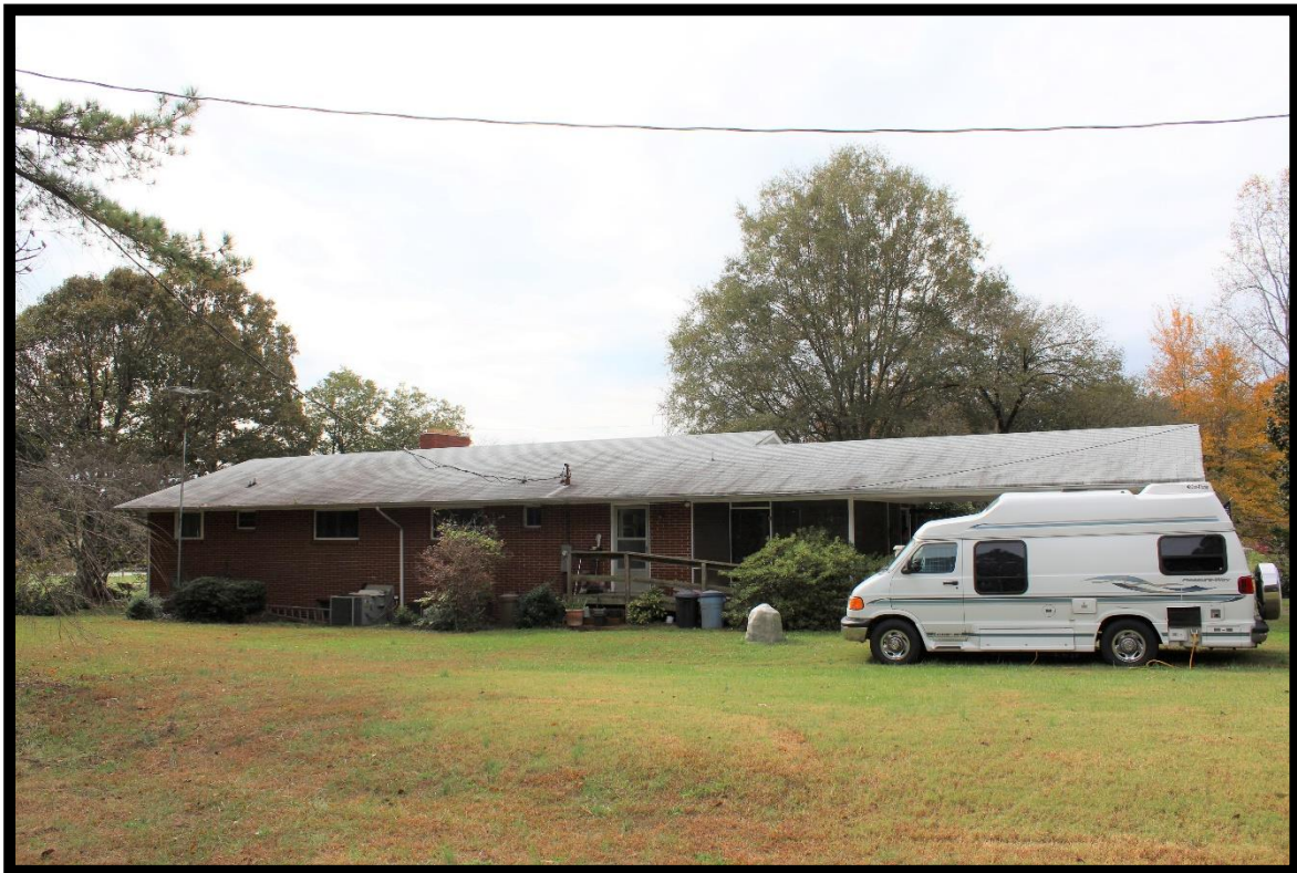
Figure 17: Chester Farmstead, Ranch Dwelling, Looking Southwest.
