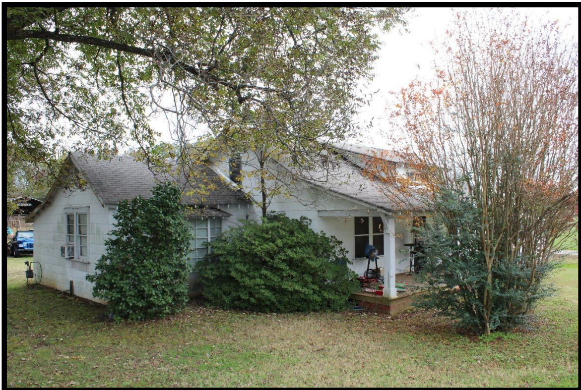
Figure 6: Chester Farmstead, Original Dwelling, Looking Southeast.
