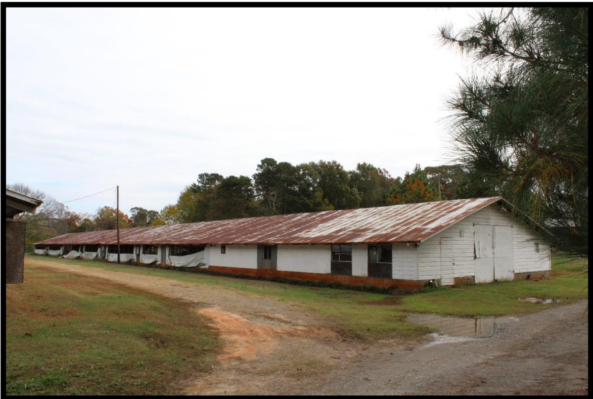
Figure 20: Chester Farmstead, Poultry Shed, Looking Southeast.
