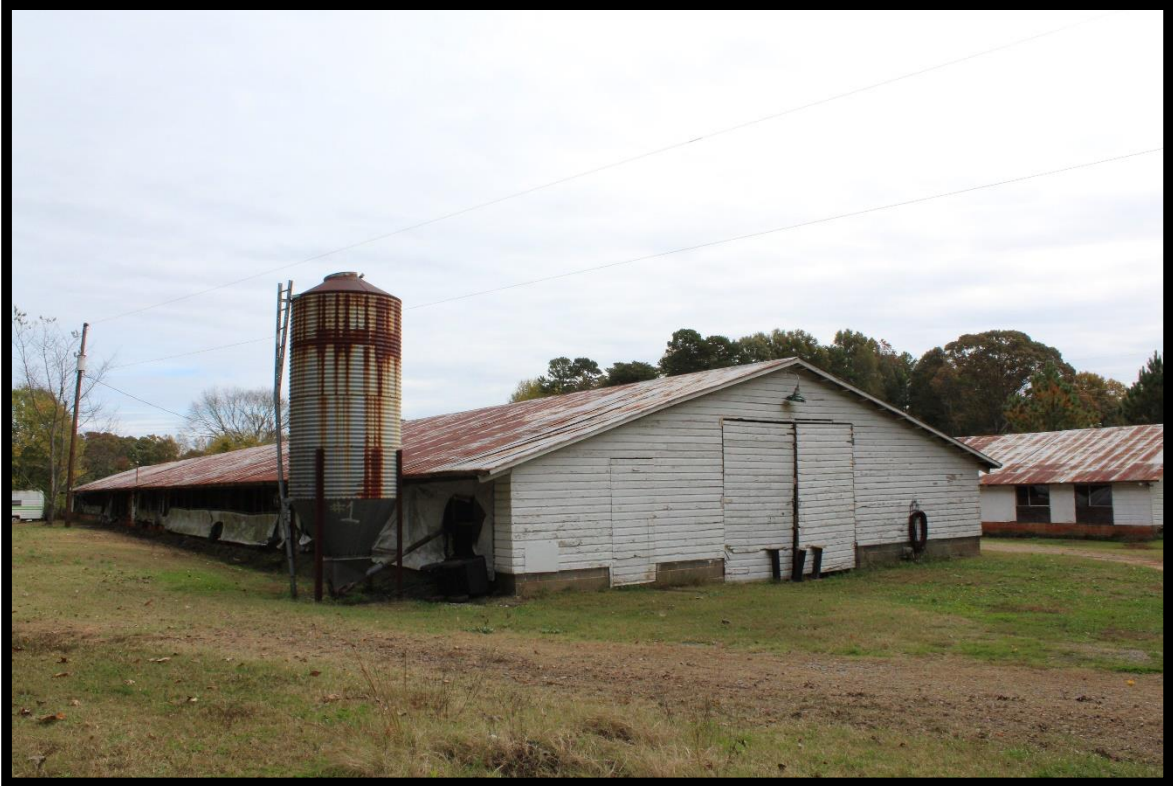
Figure 19: Chester Farmstead, Poultry Shed, Looking Southeast.
