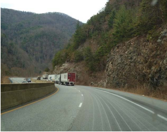
Photo 1: I-5508 Project corridor, near rock stabilization site
