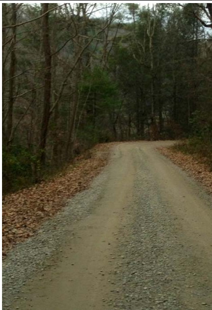
Photo 5: Typical Section of Forest Service Road 288/ Harmon Den Road
