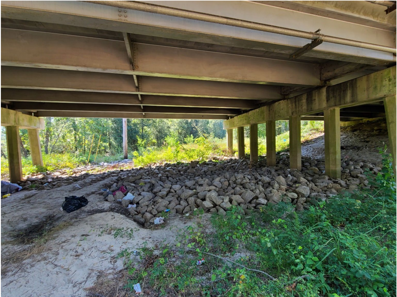
Figure C – View of bridge slope treatment and litter underneath the western side 5 th St bridge
