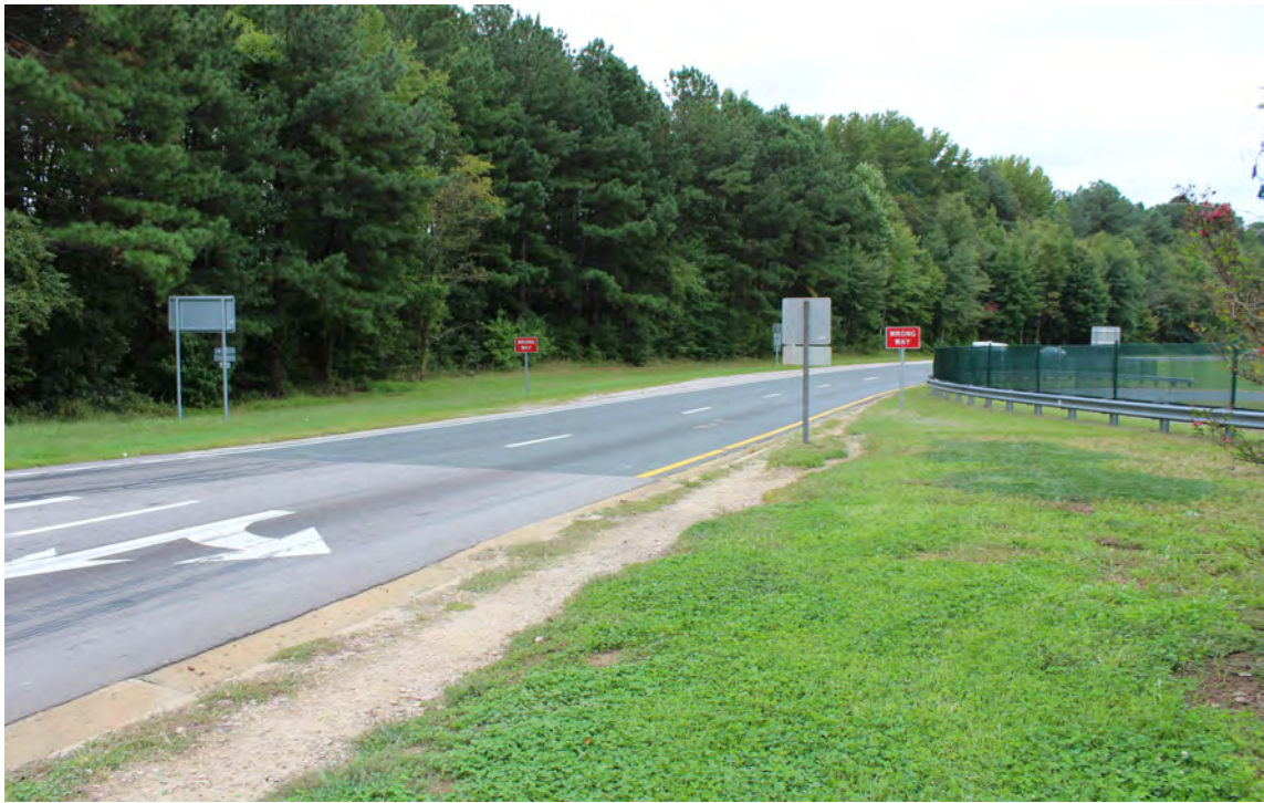
Off ramps from westbound I-40
