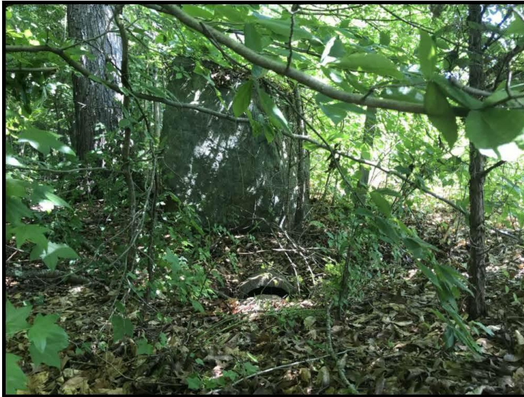
Photo 1: Location of Buried Drainpipe in Machine-Made Brick-Lined Trench, looking North from STP 3.
