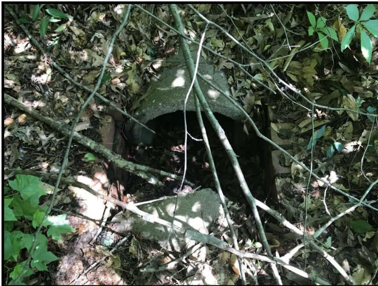
Photo 2: Closer View of Buried Drainpipe in Machine-Made Brick-Lined Trench.
