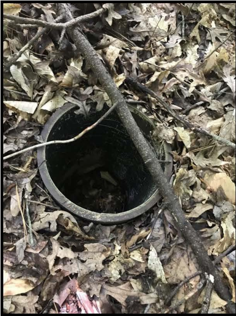
Photo 3: Close-Up View of Second Buried Pipe (Shut-Off Valve Pipe?).
