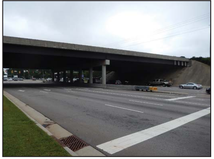
Wake Forest Road South of the I-440 Bridge, Looking North
