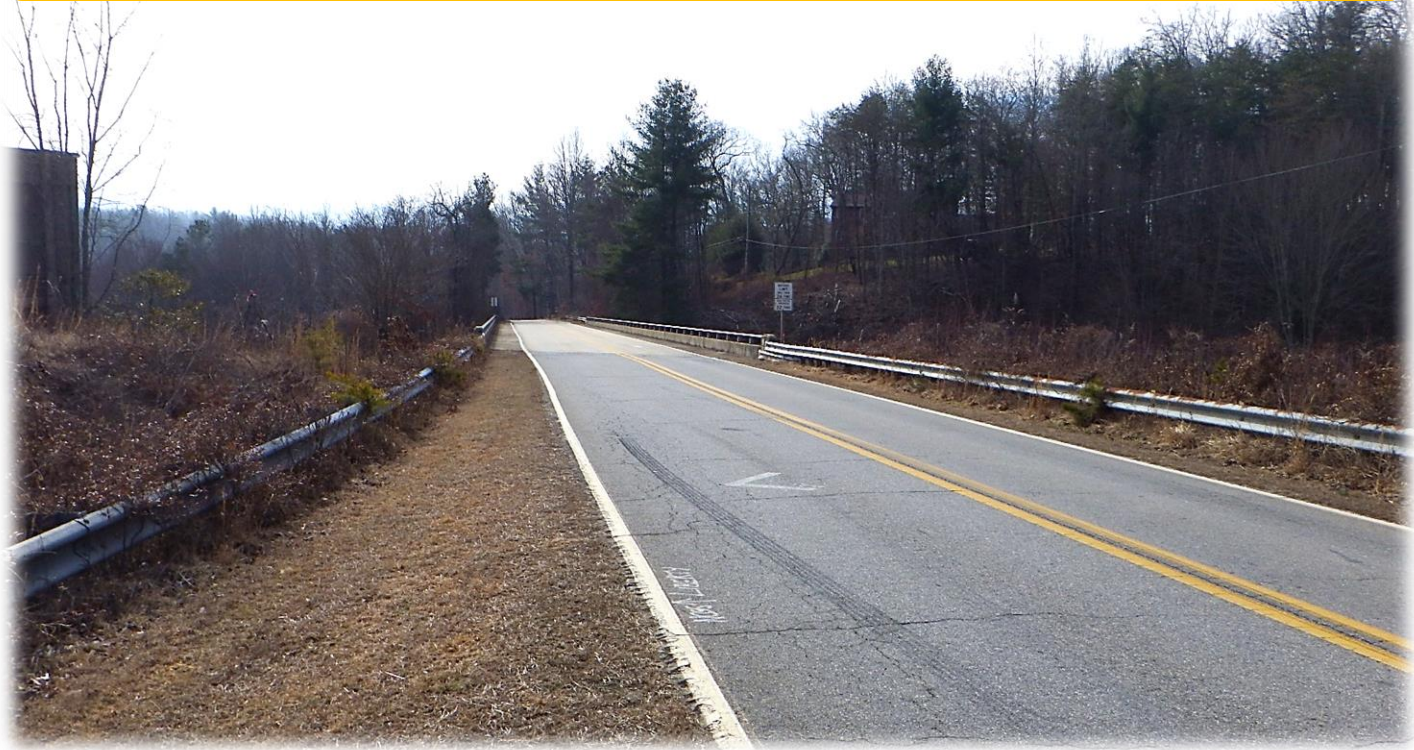
Liberty Road overpass, looking south
