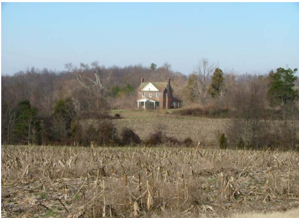
Plate 17: Looking northwest at McKee House; outbuildings at left (west) obscured by trees, and house and garage located just outside of frame at right (east); I-77 hidden by hill in distance
