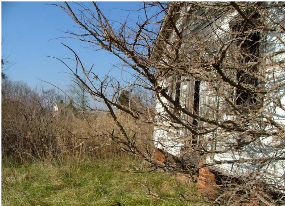
Plate 9: Looking west from deteriorated twentieth-century house toward McKee House in distance
