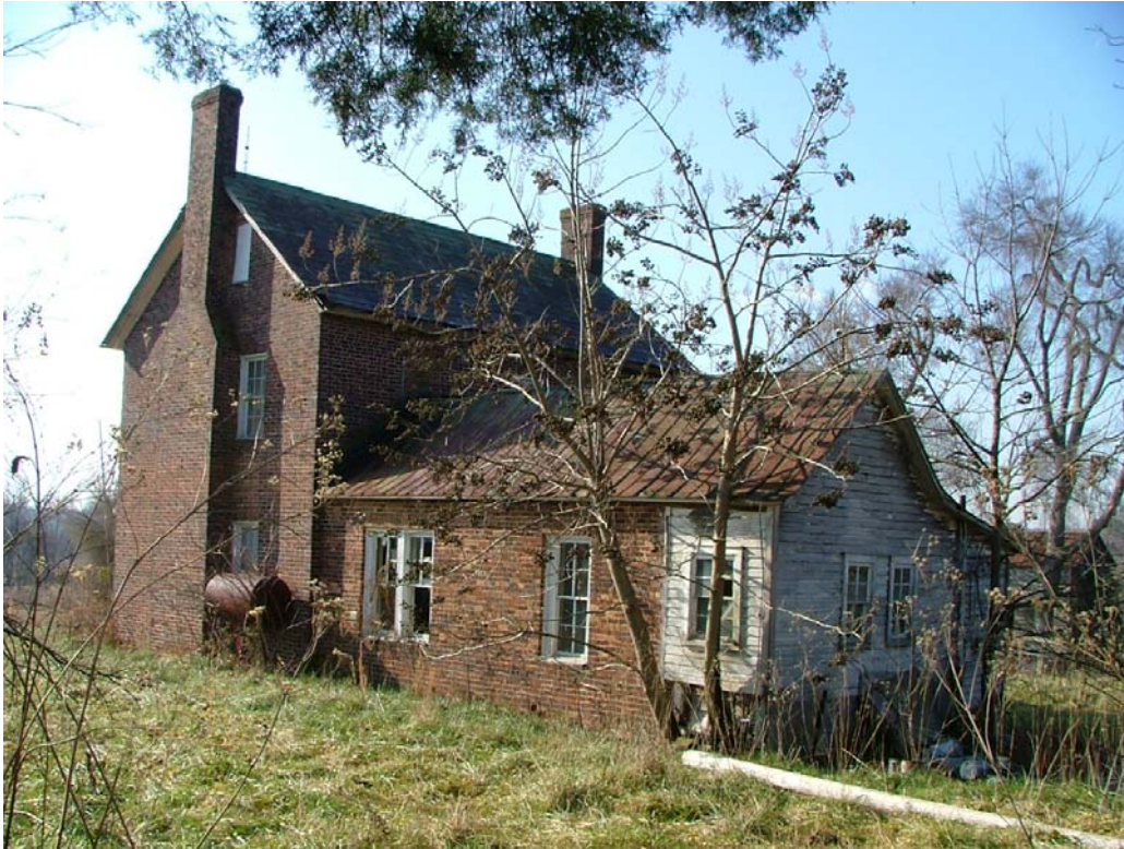
Plate 3: East side and north rear elevations of McKee House
