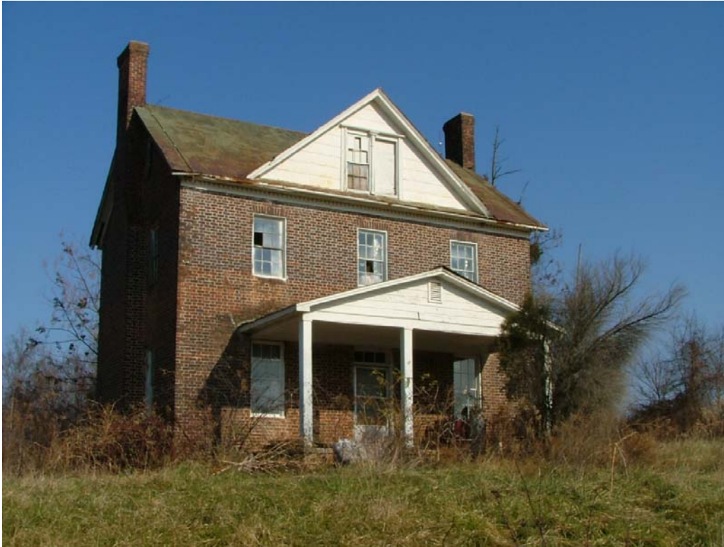
Plate 1: South front end and west side elevations of McKee House
