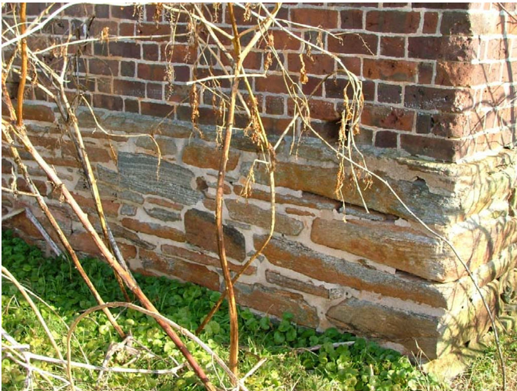
Plate 4: Detail of Flemish bond brickwork and fieldstone foundation of McKee House
