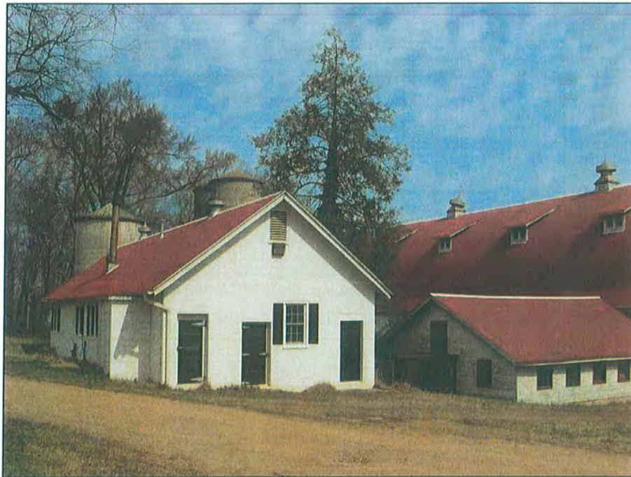
Photo of Win-Mock Farm, Dairy, S and W elevations
