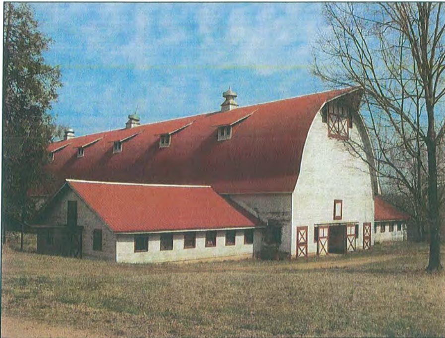
Photo of Win-Mock Farm (Property No. 2, DV 493), Main Barn, W and S elevations
