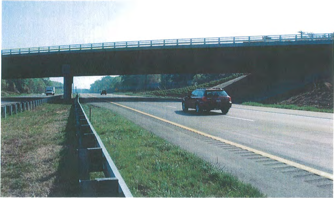
Looking East along I-40 @ Harper Road (EB) Bridge
