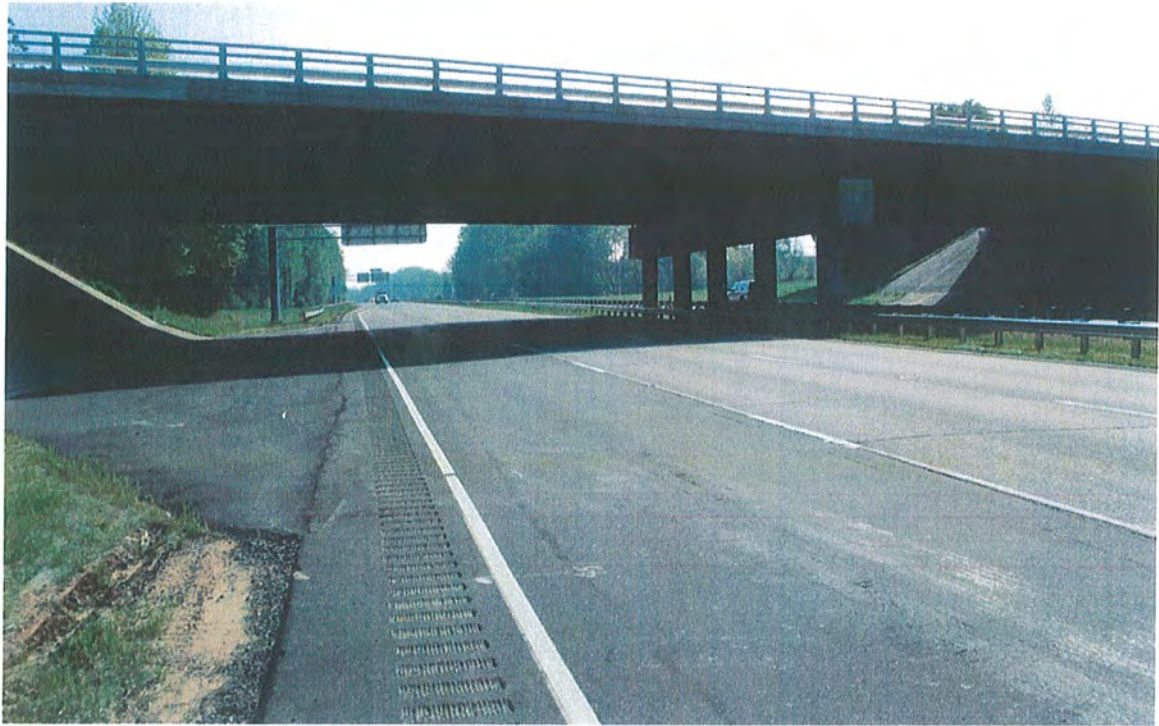
Looking East along I-40 @ NC 801 (WB) Bridge
