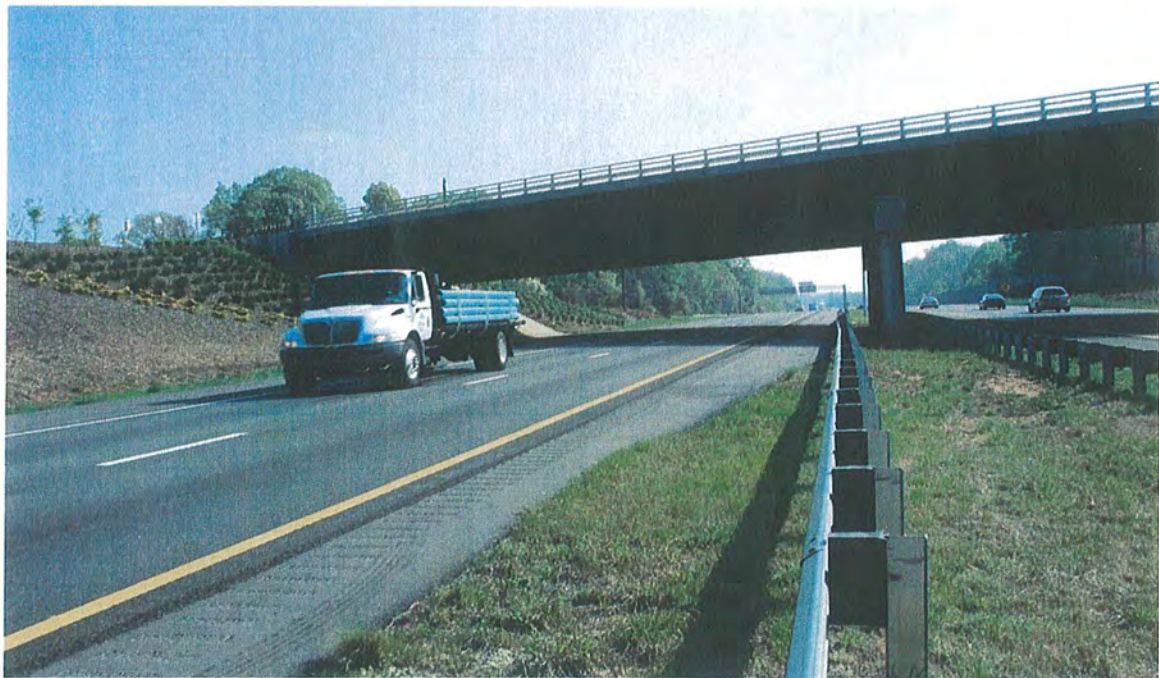
Looking East along I-40 @ Harper Road (WB) Bridge
