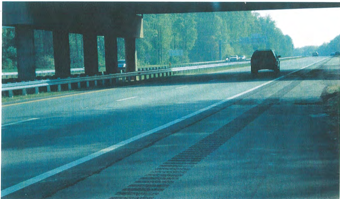
Looking East along I-40 @ NC 801 (EB) Bridge
