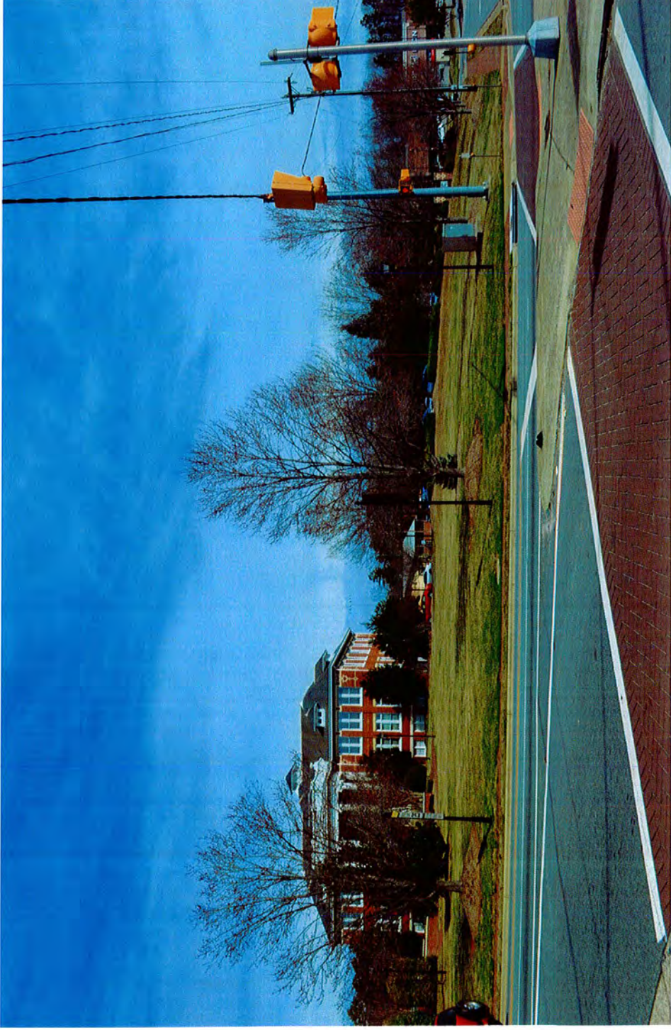
Upgraded Signal Box Northeast Corner of Ragsdale Rd and W. Main St On the Public Library Parcel
