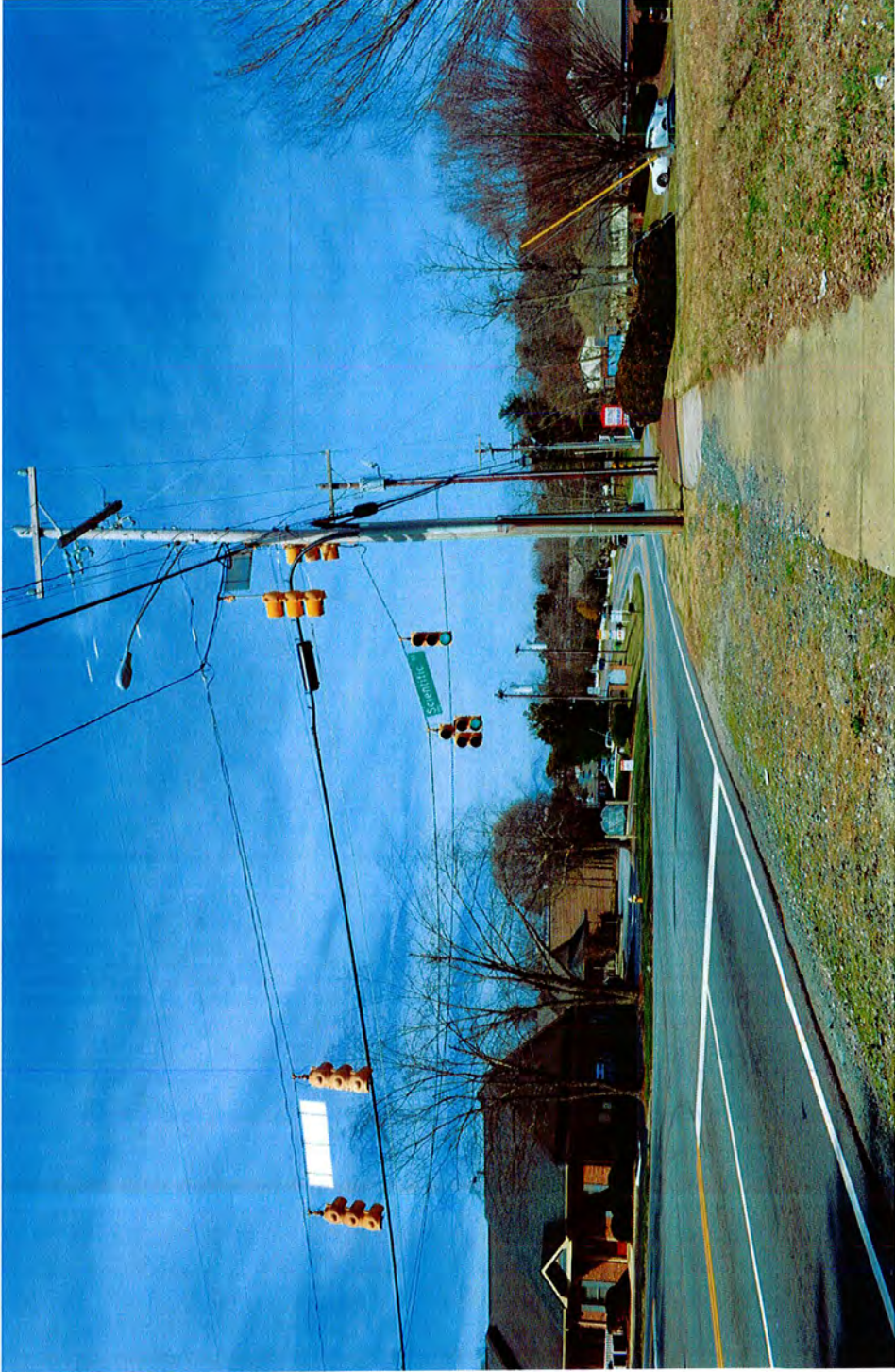
Location of Proposed Underground Cable along W. Main St. at Scientific St
