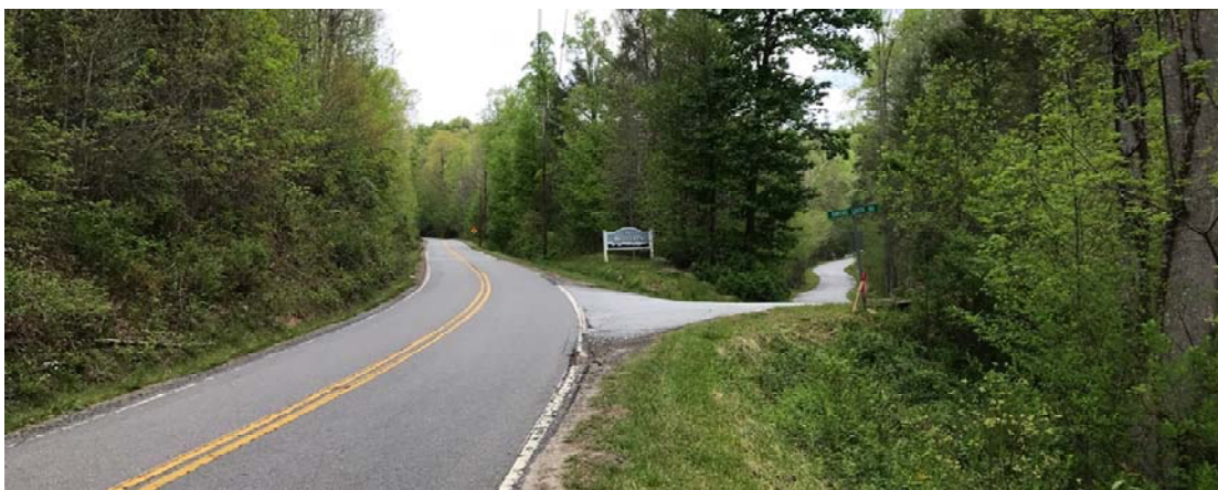
C) The NC 9 and Havens Creek Road Intersection
