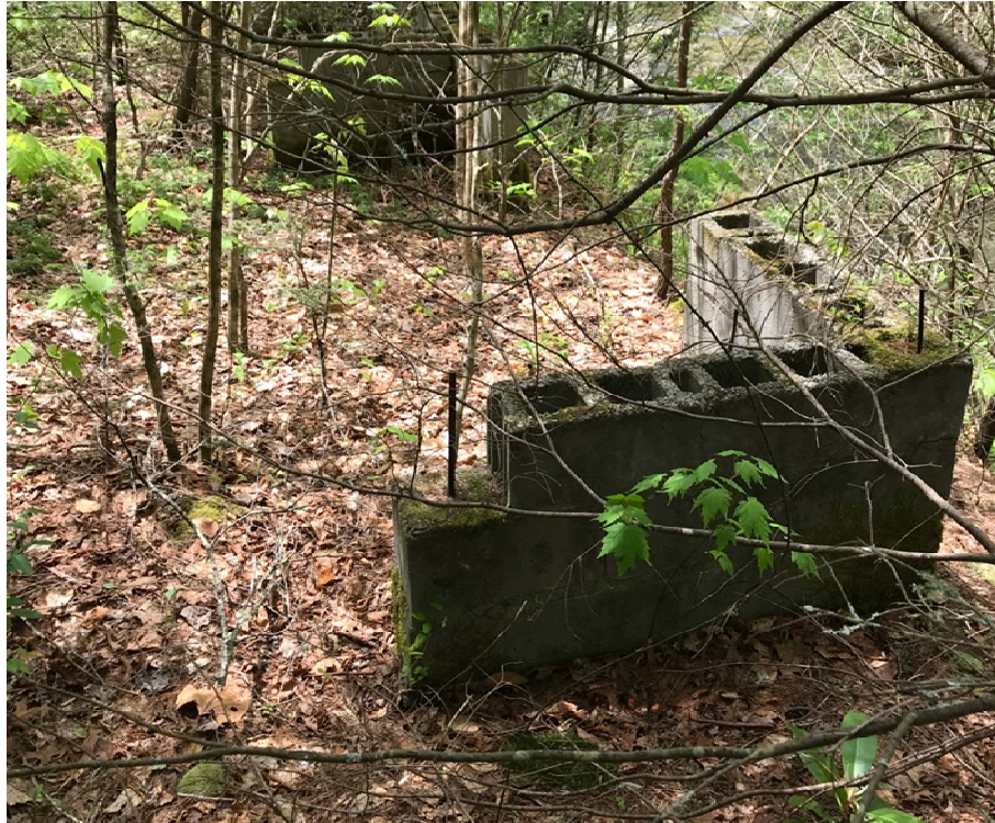
Figure 22. Partially Demolished Building Constructed in the Early 1970s
