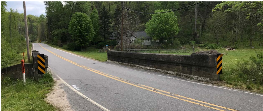
B) Bridge 79 Over the Broad River, Facing North
