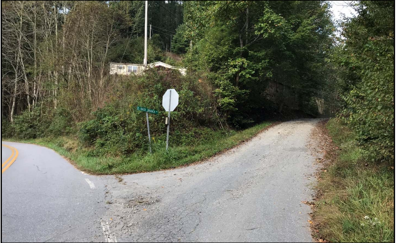
Figure 5. View of the mobile home on the graded hillside in the southwest quadrant, looking southwest.
