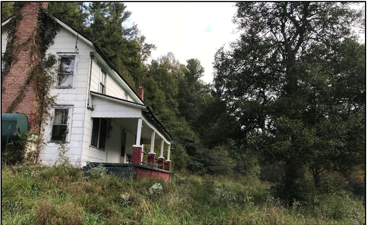
Figure 6. View of the abandon house and farm in the northwest quadrant, looking north.
