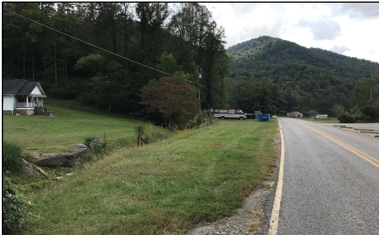
Figure 6. Area of fill between the road and Martins Creek in the southeast quadrant, looking south.
