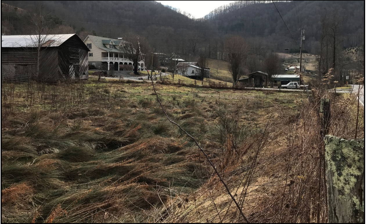
Figure 5. View of the floodplain in the northeast quadrant north of Proffitt Lane, looking south.
