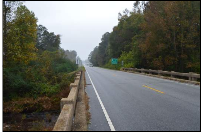
Bridge No. 246 approach facing West
