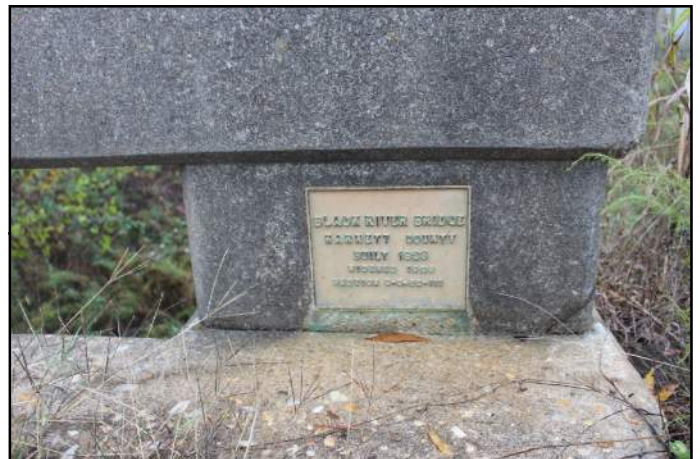
Bridge No. 246 identification plate
