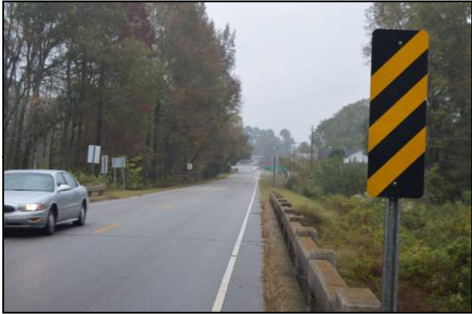
Bridge No. 246 approach facing East
