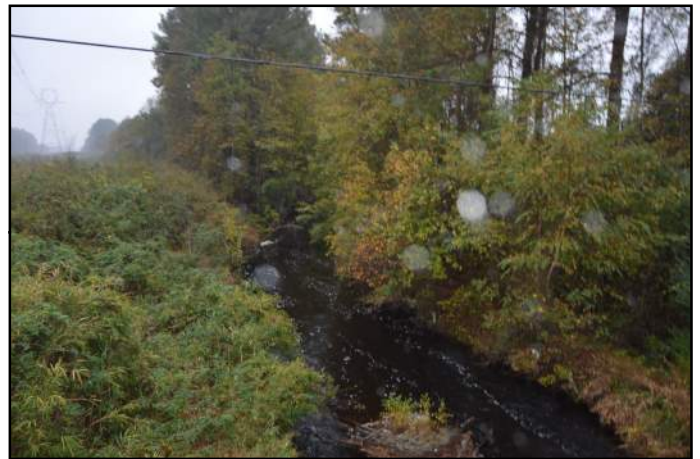
Bridge No. 246 facing South
