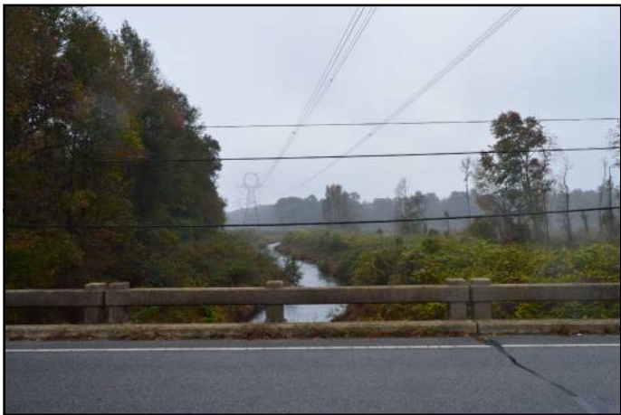
Bridge No. 246 facing North
